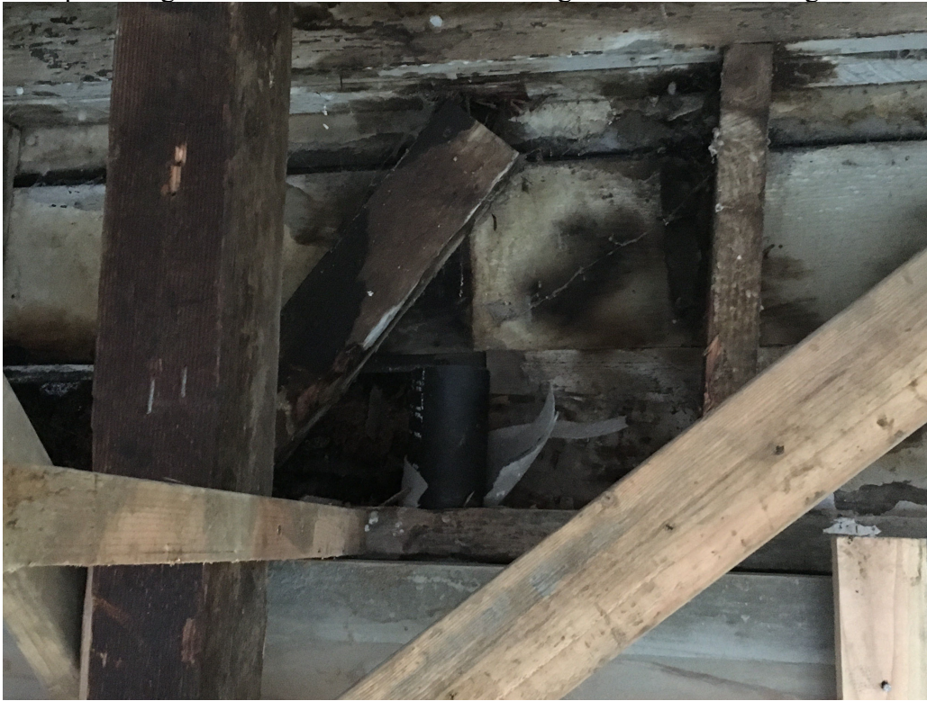
New plumbing inside of new foundation and original wall and framing:
