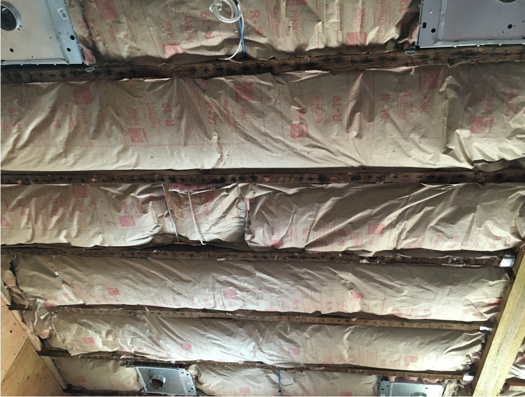
Insulation going between original ceiling joists:
