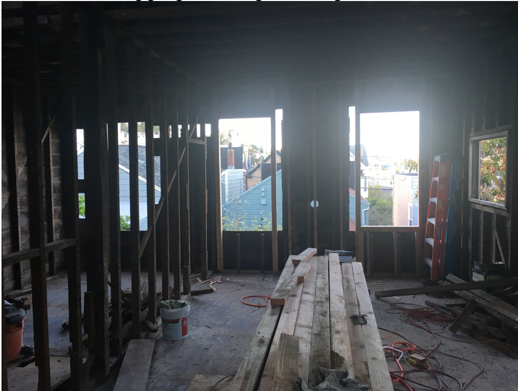
New window framing going in with original framing still intact:
