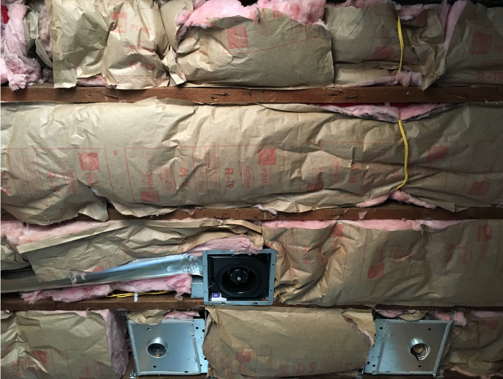
Insulation going between original ceiling joists:
