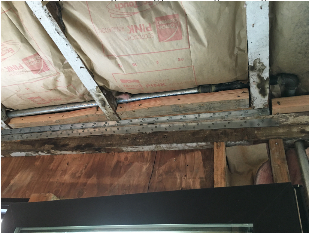
Insulation going between original ceiling joists with original framing visible:
