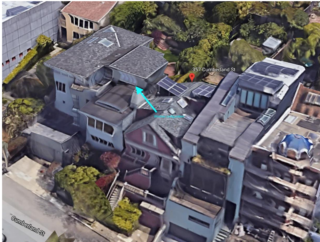
Figure 6. Distance from roof deck to north-facing front windows at 349 Cumberland
