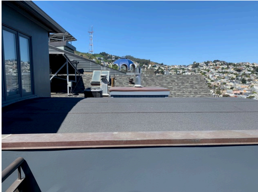
Existing roof condition from Primary Bedroom balcony showing secondary bedroom windows.
