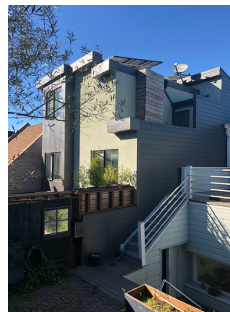
5 REAR OF NEIGH. BLDG (359 CUMBERLAND) N.T.S.
