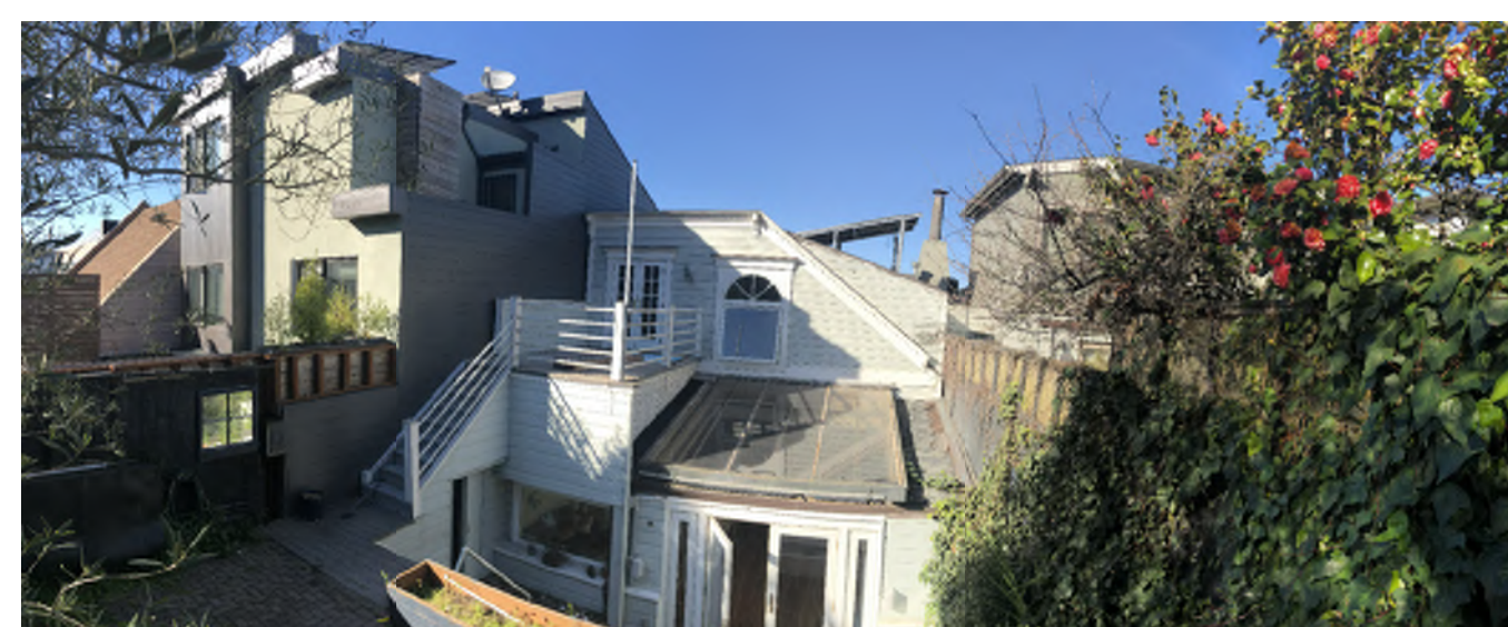
6 REAR OF SUBJECT BLDG (357 CUMBERLAND) N.T.S.
