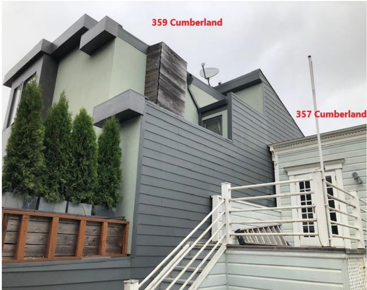
Figure 7. East façade of 359 Cumberland
