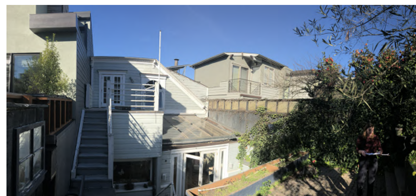
7 REAR OF NEIGH. BLDG (349 CUMBERLAND) N.T.S.
