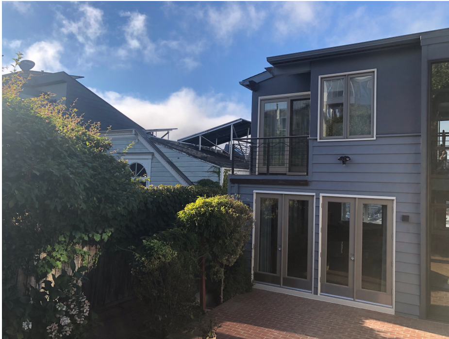
This photo shows the affected patio directly off the dining room.
