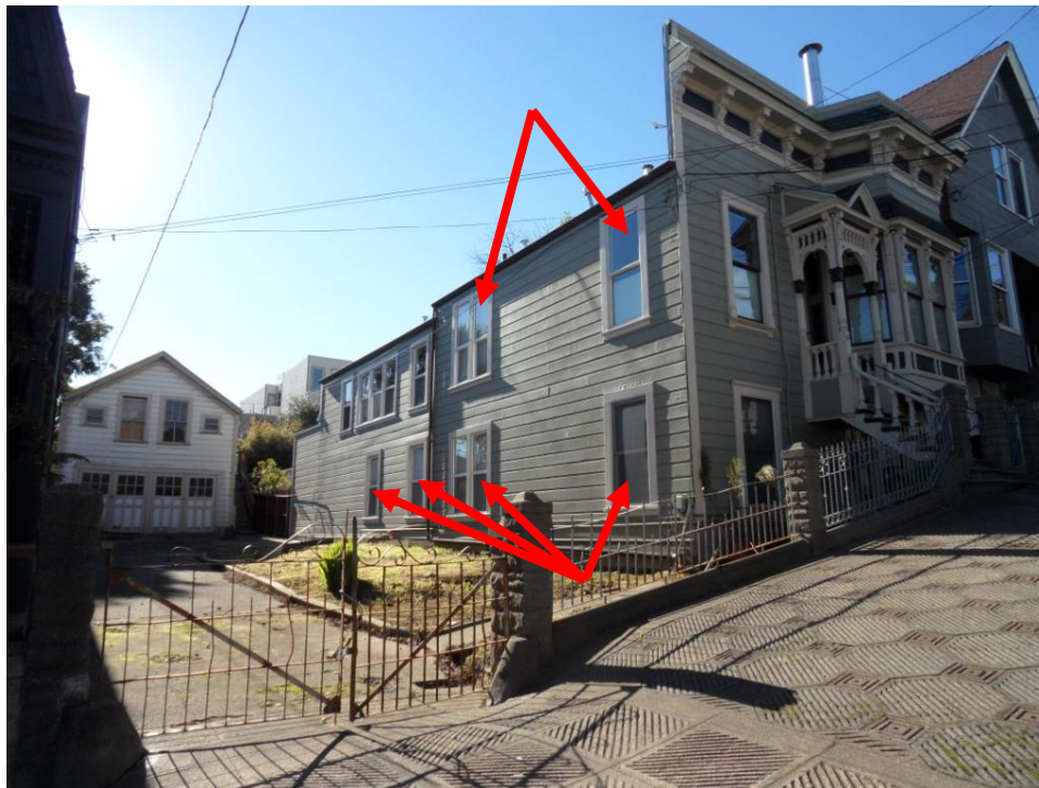
Arrows indicate windows that appear to date between 1886 and 1900.
