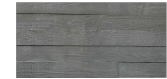
BOARD FORMED CONCRETE
