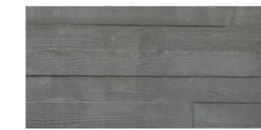
BOARD FORMED CONCRETE
