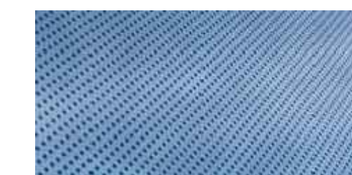
BIRD SAFETY WINDOW TREATMENTS ON 90% OF GLAZING AND ALL OF ROOFTOP GLASS RAILS
