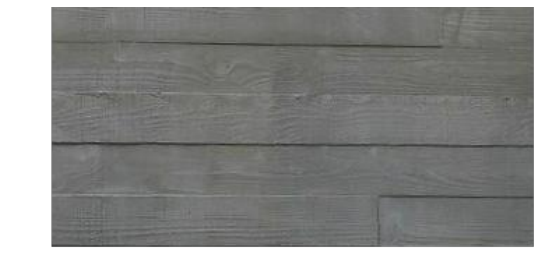
BOARD FORMED CONCRETE
