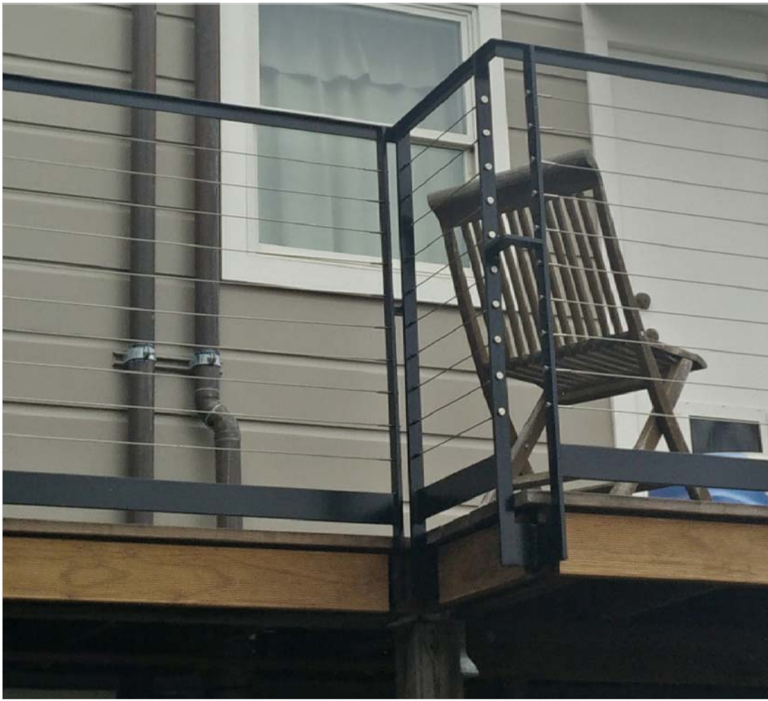
9 POWDER COATED STEEL GUARDRAIL FRAME WITH STAINLESS STEEL CABLE RAILING.
