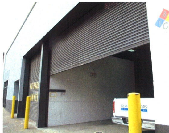
Figure 11: Vehicular entrances with metal roll-up doors.
