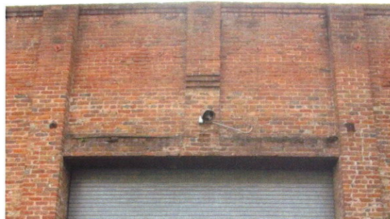
Figure 23: Brick pilasters framing garage entrance.
