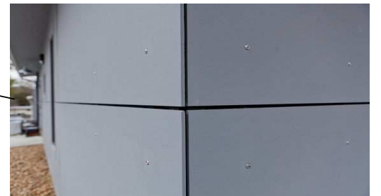
RAINSCREEN CLADDING WALL PANEL BY JAMES HARDIE REVEAL 2.0
