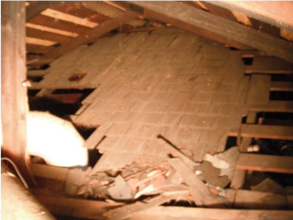
Attic showing earlier roofing systems designed as hip roof
