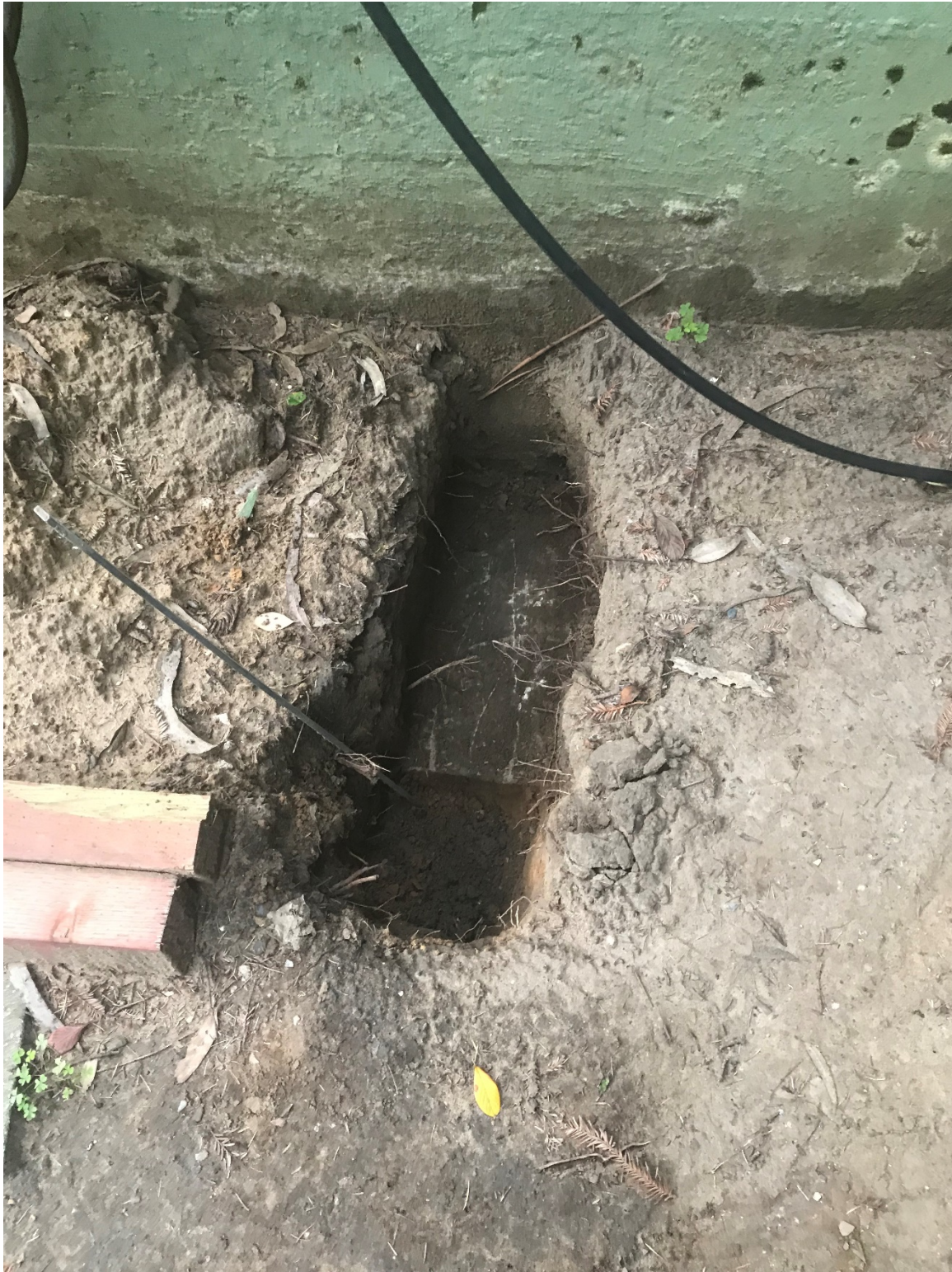
This photo shows the footing of the existing 8 foot retaining wall. It extends approximately 24 inches into the public right of way. Our excavation will be behind this wall and we believe we will be able to leave the existing footing in place.
