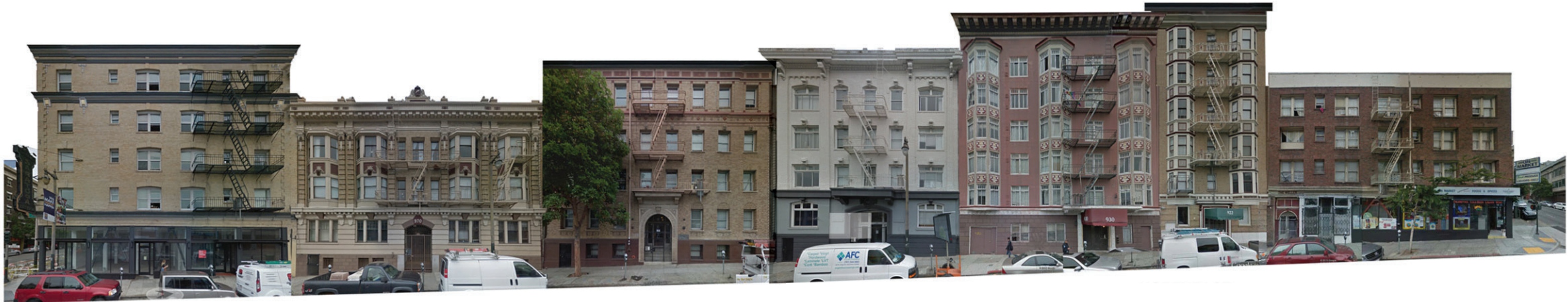
POST STREET - NORTH SIDE STREETScape
