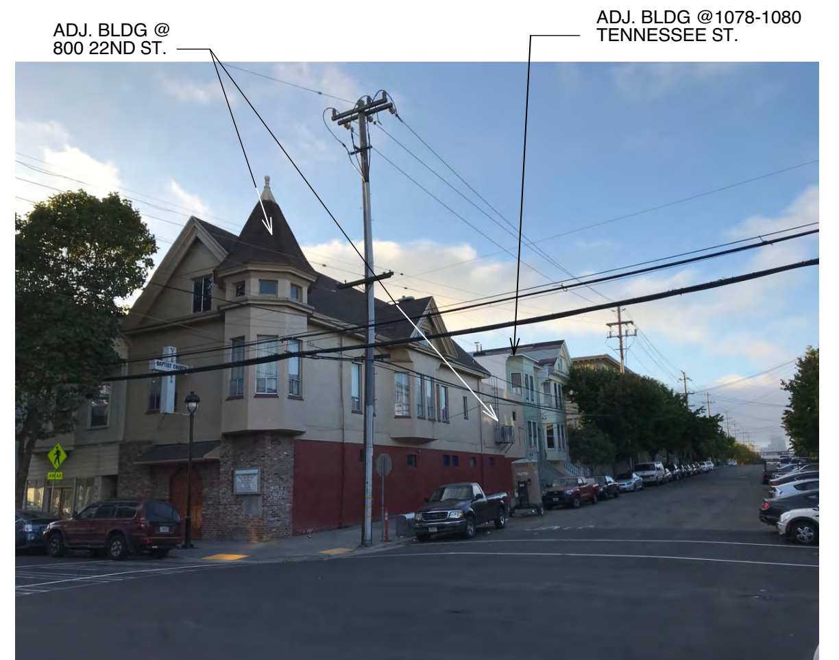
13 LOOKING NORTH - WEST
