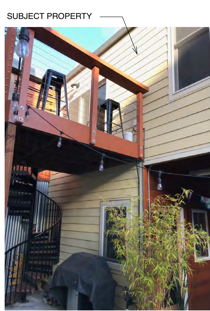
3 LOOKING NORTH - EAST
