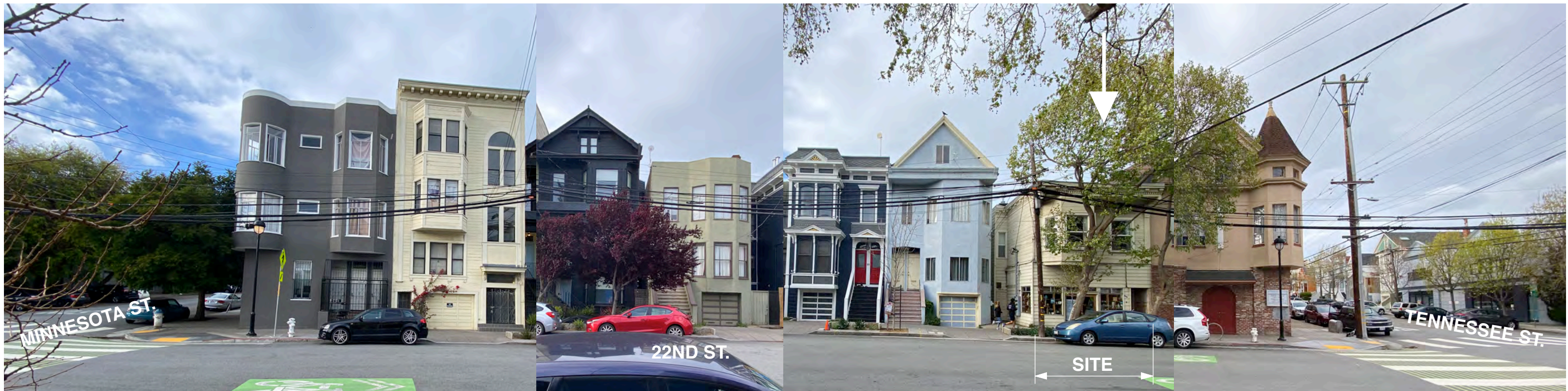
N 22nd STREET / North Side - 800 block
