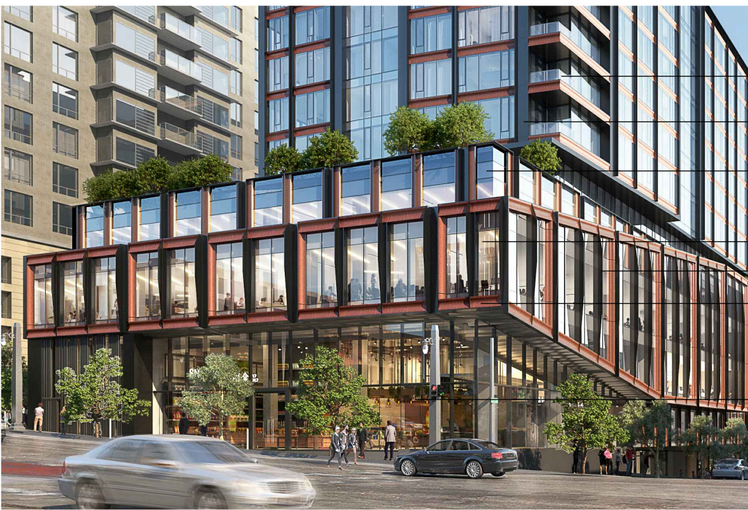
IMG. 1 - VAN NESS AVENUE & POST STREET
