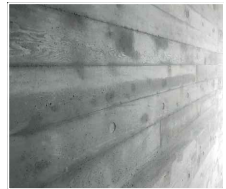
BOARD FORMED CONCRETE
