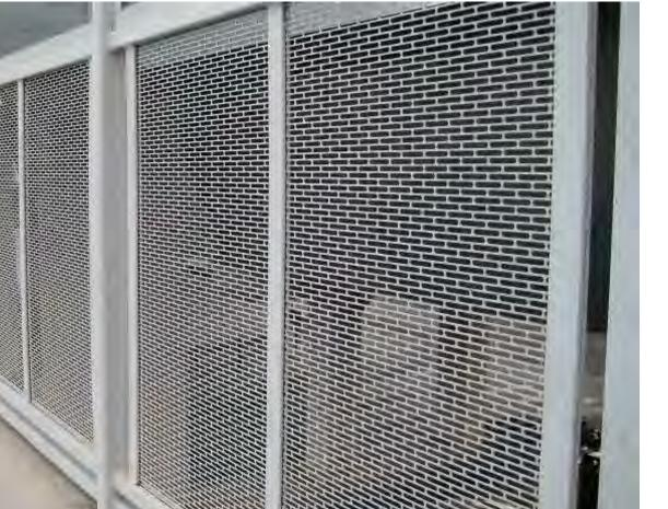
PERFORATED METAL PANEL / GUARDRAIL
