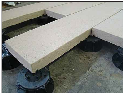
PRECAST CONCRETE PANELS ON PEDESTALS
