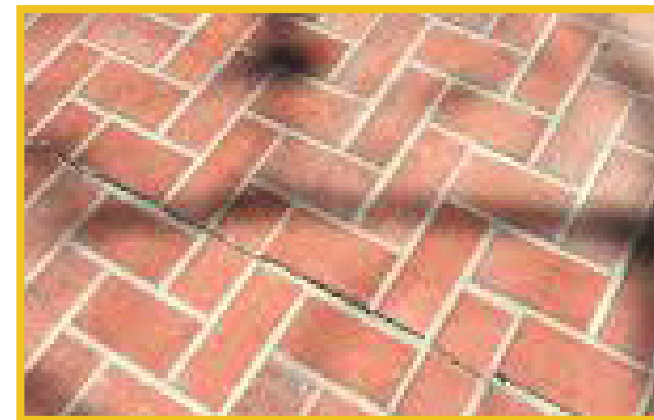
MARKET STREET STANDARD PAVING
