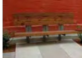
CUSTOM WOOD BENCH WESTERN RED CEDAR WITH PRIMED AND PAINTED GALVANIZED STEEL BRACKETS AND ARMRESTS
