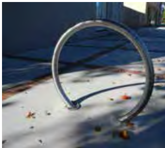
BIKE RACKS (3 EACH) SURFACE MOUNTED WITH STAINLESS STEEL FINISH
