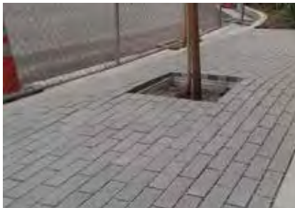
CONCRETE UNIT PAVING IN STREET TREE WELLS 6" X 12" GROUND FACE, THROUGH COLOR WITH 1/4" SPACERS
