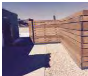
10' HIGH UTILITY SCREEN WESTERN RED CEDAR WITH PRIMED AND PAINTED GALVANIZED STEEL FRAMING & GATE MAINTENANCE
