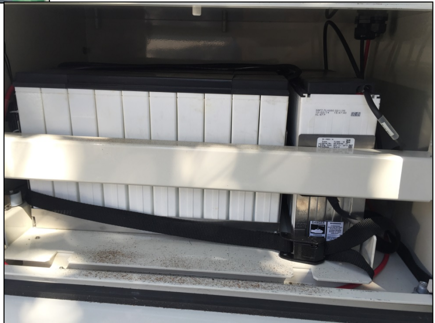
Batteries inside cabinet used to provide backup power to operate WTS facility, in case of power outage
