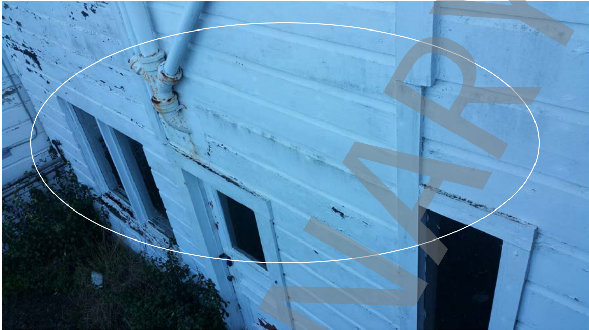
Photo # 14: Improper flashing, improper waterproofing detailing, rot, peeling lead paint at the back of the house.
