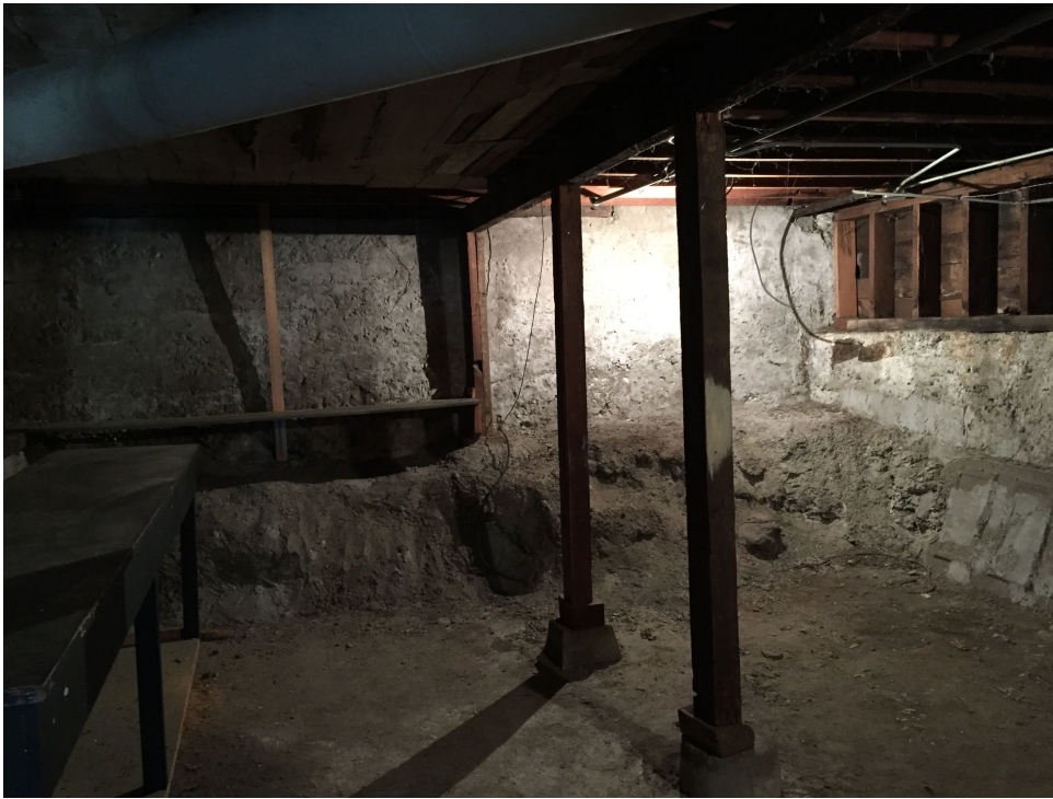
Photo 6. This photo shows the retaining wall at the front property line. Note that the original wall only extends down about 1/2 to 2/3 of the current total headroom depth. The bottom portion is crudely excavated and covered with rat slab, and provides no confinement or support of the base of the original retaining wall.
