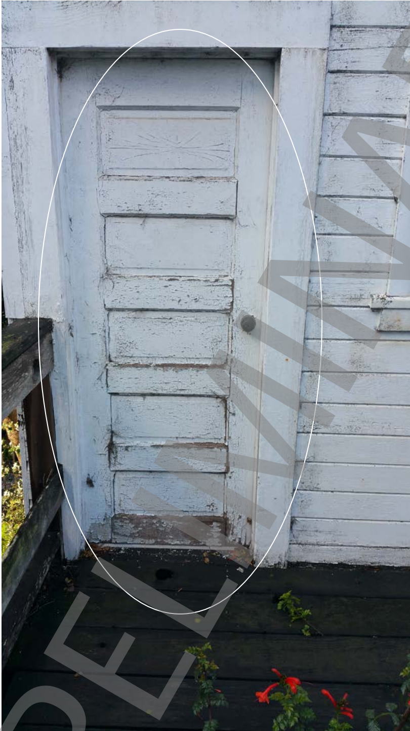
Photo # 18: Rotten broken door, with peeling lead paint, at back structure.
