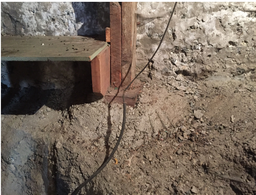
Photo 7: This photo shows a post supporting the central bearing line adjacent to the front retaining wall. Note how the support at the base of this post has been built up with concrete on the surface of the excavated face. This suggests that the original support for this post was also undermined through the process of the secondary excavation.
