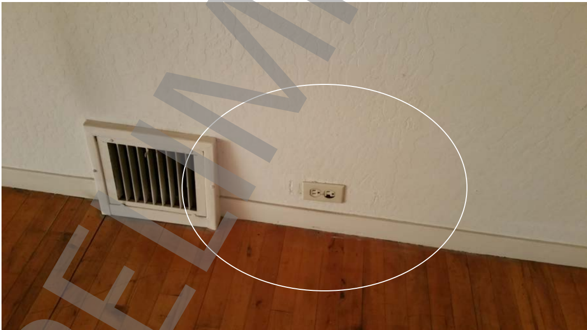
Photo # 11: Broken and improperly placed electrical outlets, and other fixtures.
