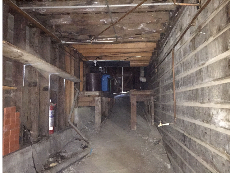
Photo 14: This image, taken farther down the driveway from the previous one, shows the floor framing in the kitchen area. Note that the framing in this area includes newer, dressed lumber, as well as framing that is obviously older (foreground). In addition, the property line post and beam support at the top of the driveway has been replaced with a studwall, albeit one that does not have exterior siding. Once again, the siding from the adjacent building can be seen beyond, and there is no separation between buildings.
