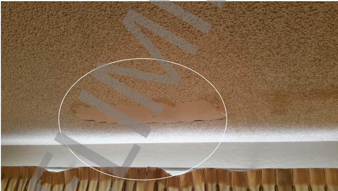
Photo # 3: Leaking roof in living room and dining room.
