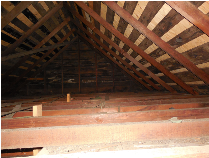
Photo 22: This photo shows the gable roof over the original section of the building. Note the long spans on the rafters, with no collar ties or kickers. Note also the 2x4 stickers hanging down to support the dropped ceiling below.
