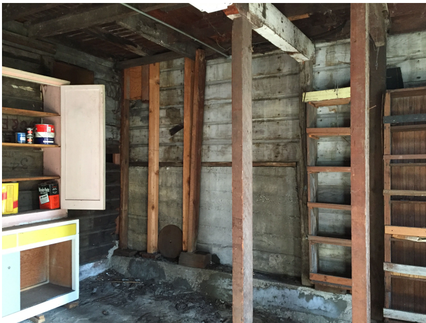
Photo 19: This photo shows the south property line, where the floor framing runs parallel to the property line and there is no studwall at all. The siding that can be seen here is on the adjacent building. Note the three sections of floor framing, which use members of different sizes. In particular, note how the central section is supported on the edge of a 2x member, which is laid on the flat on top of the beam. This area is located between gridlines 7 and 8.
