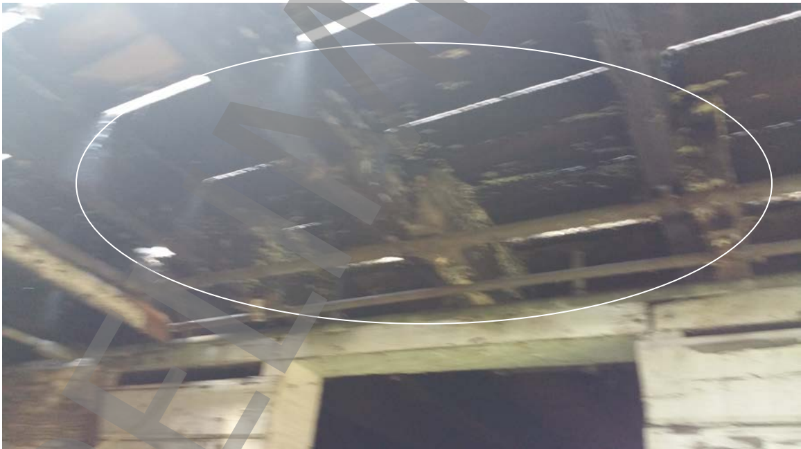
Photo # 26: Rotten framing and missing siding and waterproofing.
