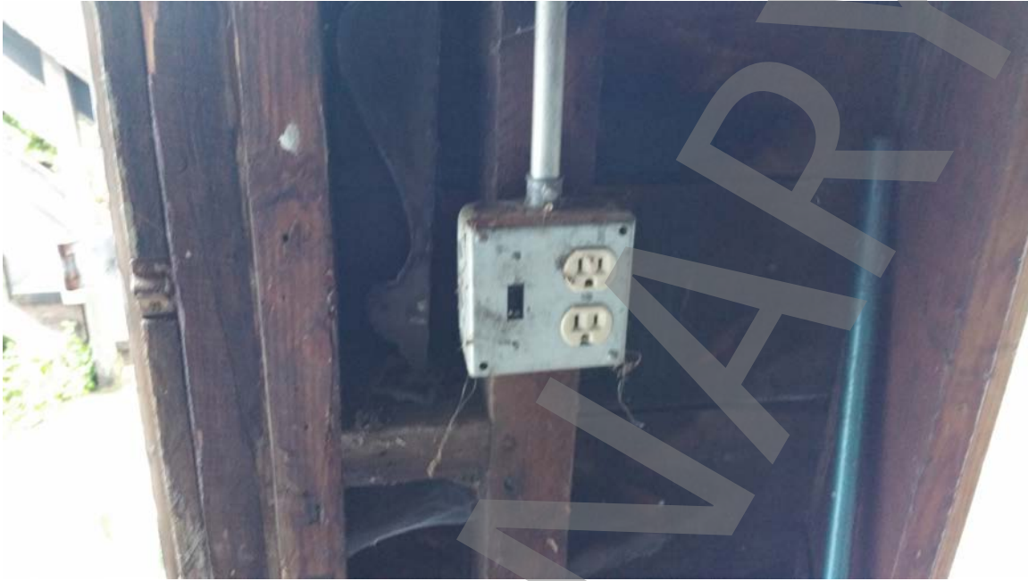
Photo # 39: Broken and improperly installed electrical throughout.
