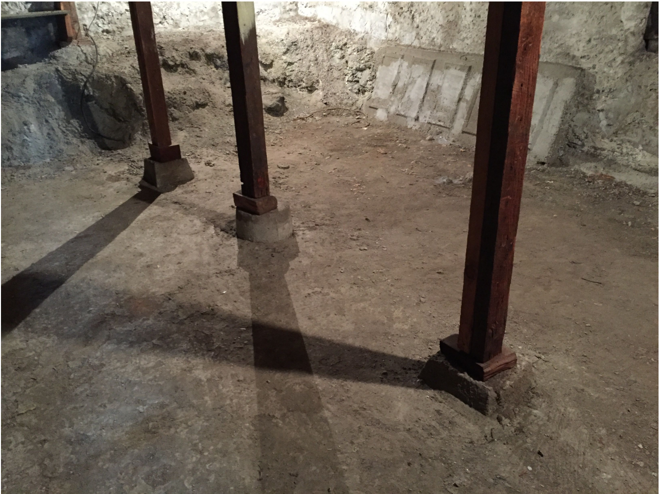
Photo 11: This photo shows the pad footings for the posts that support the central bearing line. Note that none of these footings are the same, which one would expect if they were all placed at the same time. Also note that they are all shored up with large blocks at their base. While it is typical to place a wood pad at the base of the post to separate the post end grain from direct contact with the concrete, large blocks like this would be atypical. This condition also lends support to the notion that the original floor was excavated below its original level. In addition, they are undersized for the loads they carry, and therefore they cannot adequately spread their point loads over a large enough bearing area. They likely lack any embedment, and there are no physical connection between the posts and their support footings.
