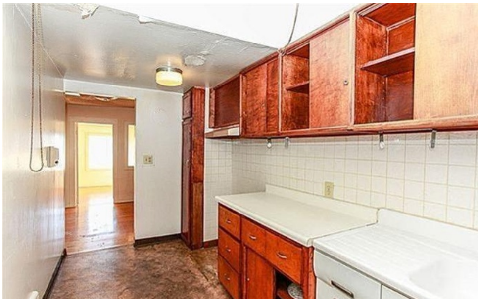
Photo 7: This photo shows the kitchen area, which was also created by infilling over the driveway at the north side of the building. Note the change in ceiling height at the back of the room. The majority of the roof over the kitchen is a continuation of the roof over the elevated bedroom at the front of the building.
