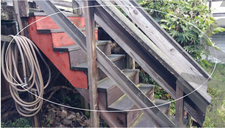
Photo # 29: Stair rotten, stringer cut, very steep, no handrail, holes in guardrail, not to code.
