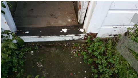
Photo # 29: Stair rotten, stringer cut, very steep, no handrail, holes in guardrail, not to code.
