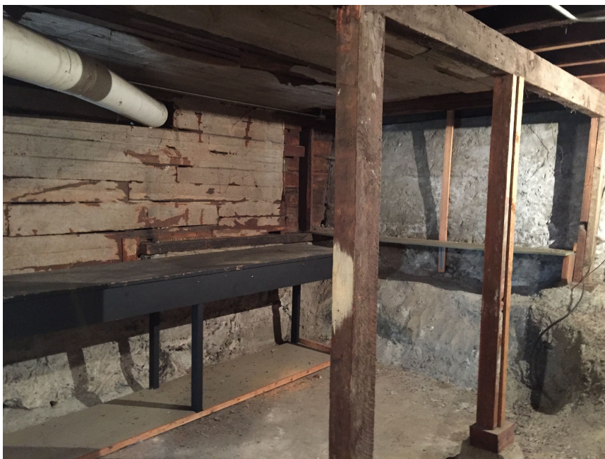
Photo 24: This photo shows the central post and beam system at the original section of the building. The narrow building, combined with the central support renders the floor joists adequate, but the beam does not meet the demand imposed by the loads required by the code in effect at the time of original construction. This beam needs to be replaced.
