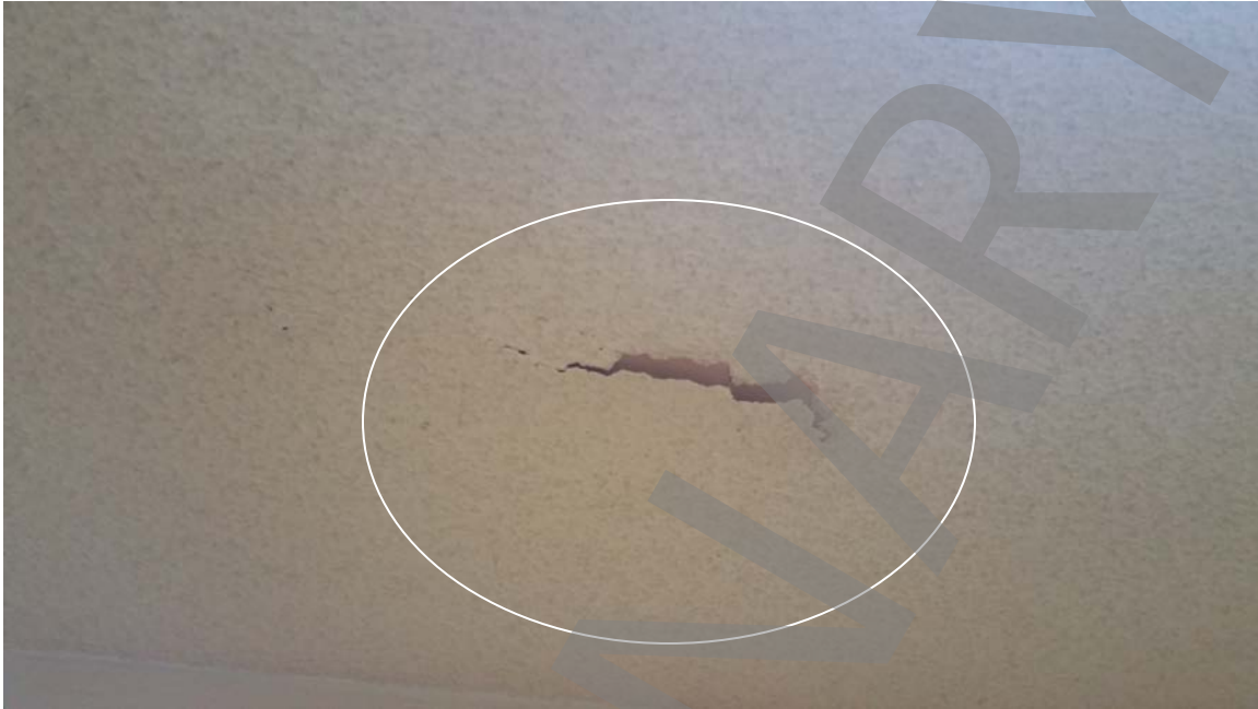
Photo # 12: Flaking and peeling asbestos finish in dining room.
