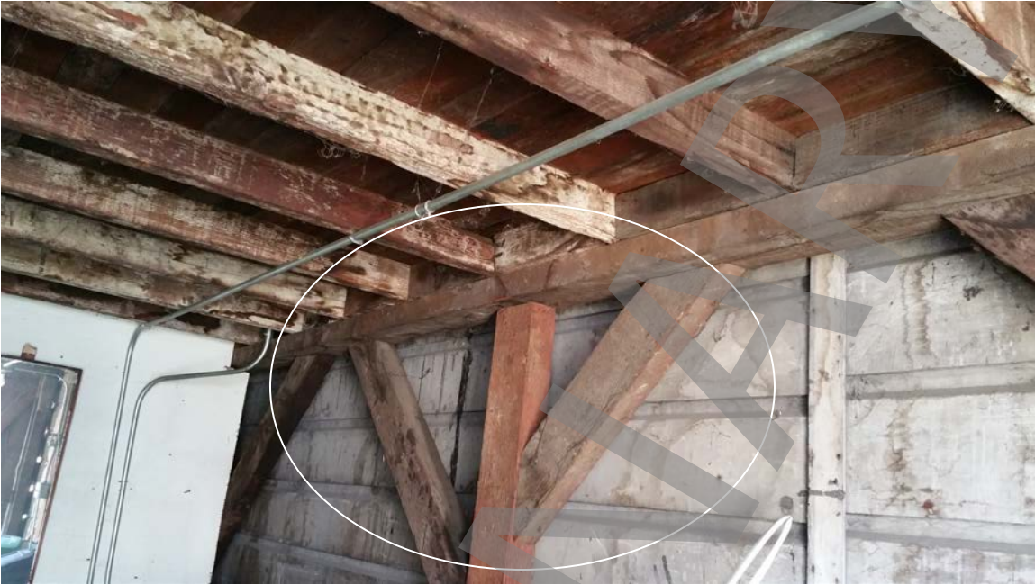
Photo # 43: Undersized floor joist. No exterior side walls on lower story, typical, ( this is the neighbor's siding.) Inadequate seismic posts, bracing and detailing.
