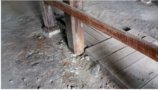
Photo # 35: Improper wood separation in area without weather protection, beetle infestation, rot.
