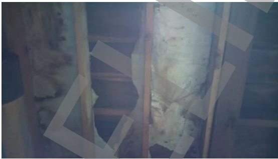
Photo # 38: Damaged moisture barrier, or no exterior wall, where occurs, typical.
