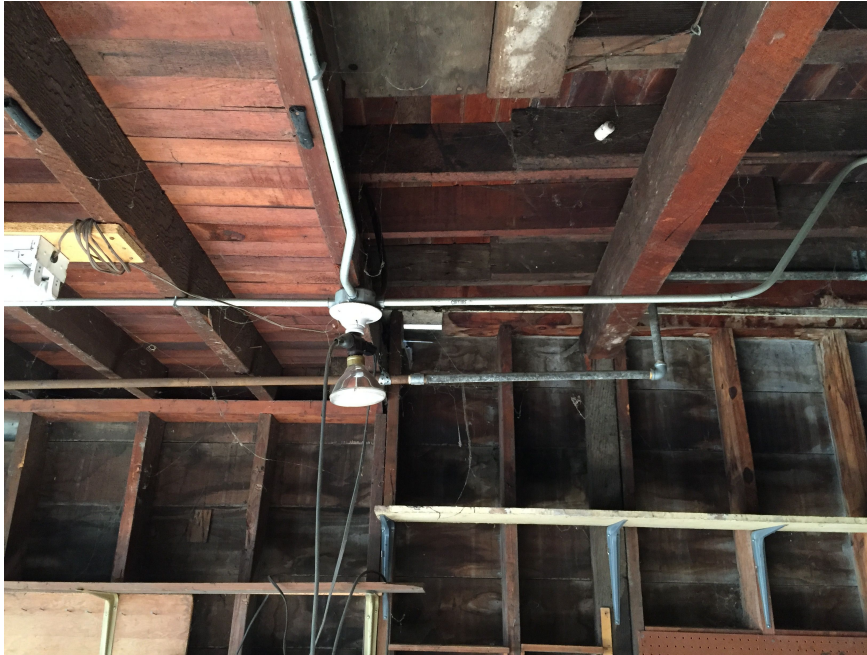
Photo 17: This photo shows the floor framing above the north property line at the rear from the previous photo. Note the three distinct sections of floor framing—left, middle, and right—along with changes in framing direction. The beam is at gridline 7. The framing at the left is somewhat mysterious, because it appears that there are two levels of floor framing, one on top of the other. The area corresponds to Bedroom 3, and there is no change in elevation between the Dining Room and Bedroom 3.
