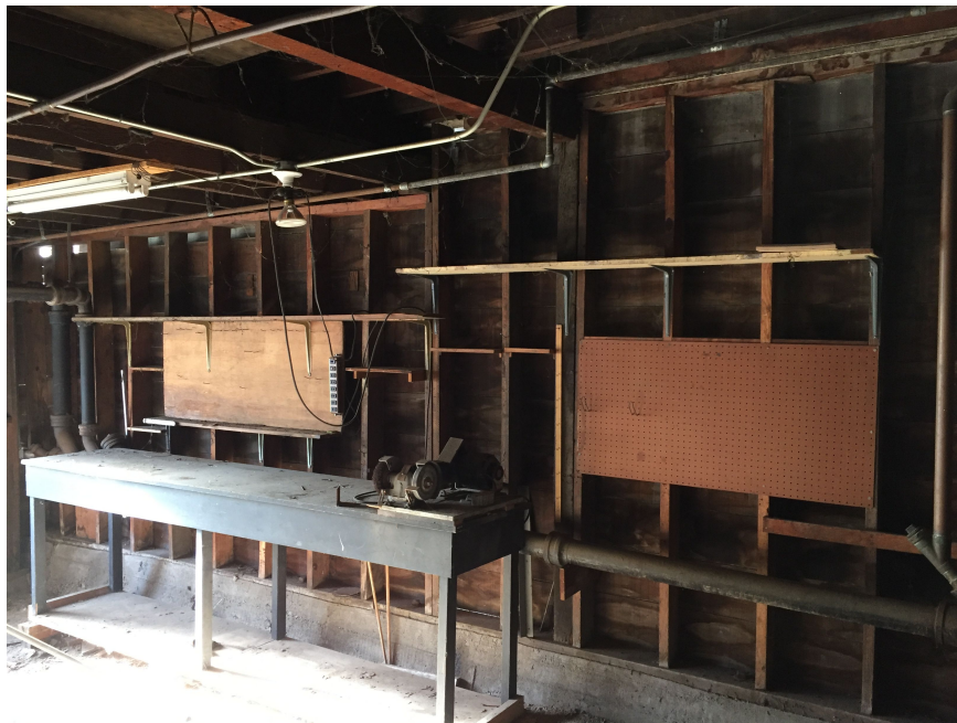
Photo 16: This photo shows the continuation of the north property line wall. Here the construction is newer, with dressed lumber and exterior sheathing, but no evidence of a permit.
