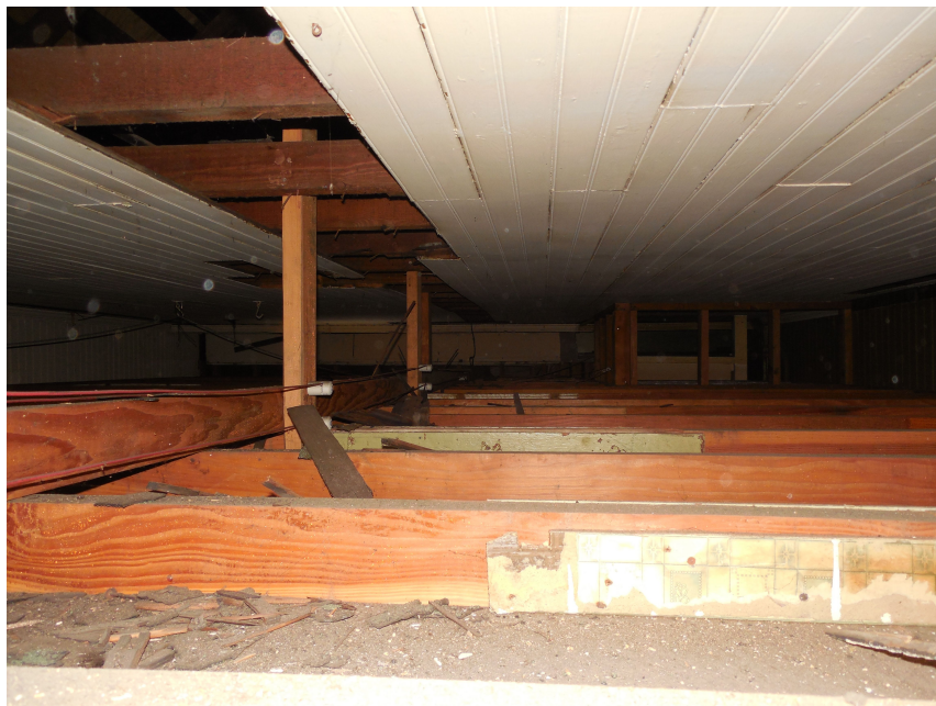
Photo 23: This photo shows the interstitial space between the original ceiling, clad in T&G beadboard, and the dropped ceiling.
