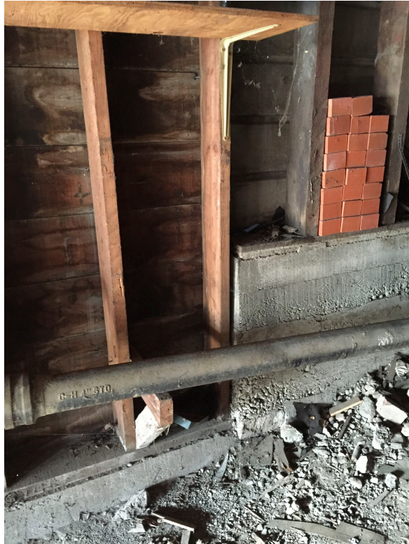
Photo 15: This photo shows a transition between newer and older construction along the north property line. Note the older framing to the right, with no exterior siding. To the left is a section of newer construction, which is marked by the dressed lumber and the exterior siding. Also note the change in the footing at this location. This transition occurs at roughly gridline 5, which marks the rear extent of the original structure. The older section represents the driveway area that could have been potentially been covered as part of the 1924 permit. If that were the case, then the remaining construction beyond, which clearly newer, could not have been permitted.
