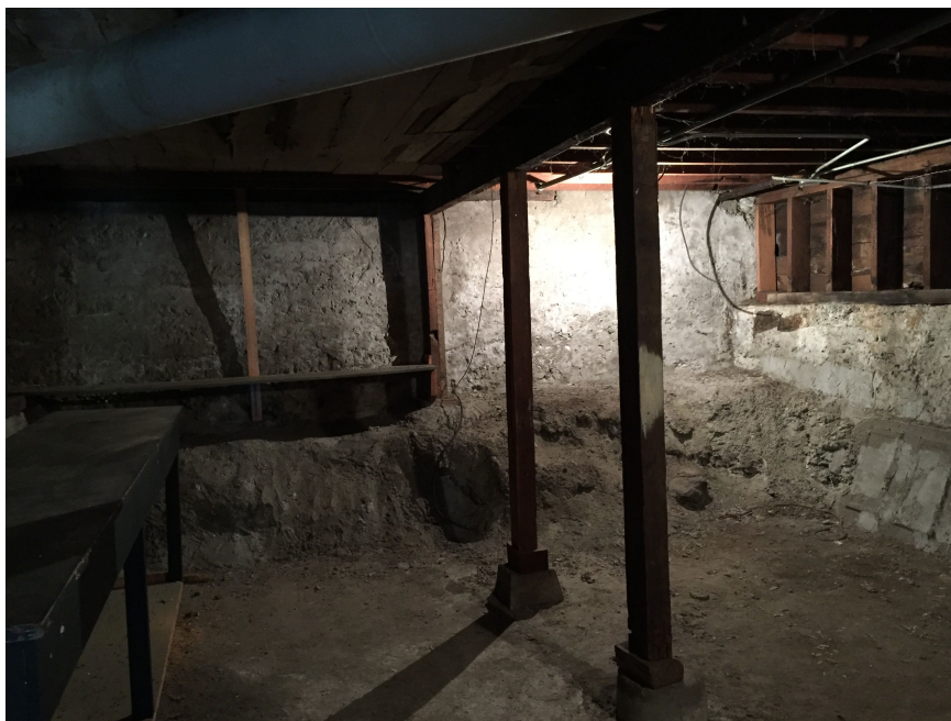
Photo 10: This photo shows the basement area under the original building. Note the retaining wall at the back, which has been undermined in order to create more headroom at the rear of the storage area.
