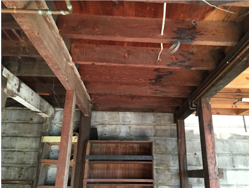
Photo 19: This photo shows the south property line, where the floor framing runs parallel to the property line and there is no studwall at all. The siding that can be seen here is on the adjacent building. Note the three sections of floor framing, which use members of different sizes. In particular, note how the central section is supported on the edge of a 2x member, which is laid on the flat on top of the beam. This area is located between gridlines 7 and 8.
