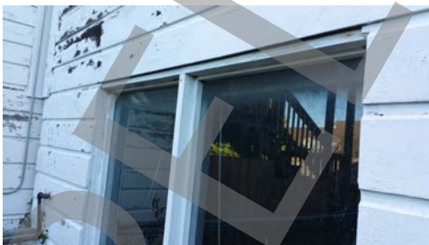
Photo # 30: Rot, improperly built waterproofing details, peeling lead paint.
