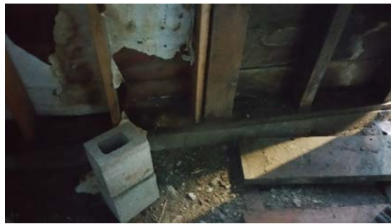
Photo # 38: Damaged moisture barrier, or no exterior wall, where occurs, typical.
