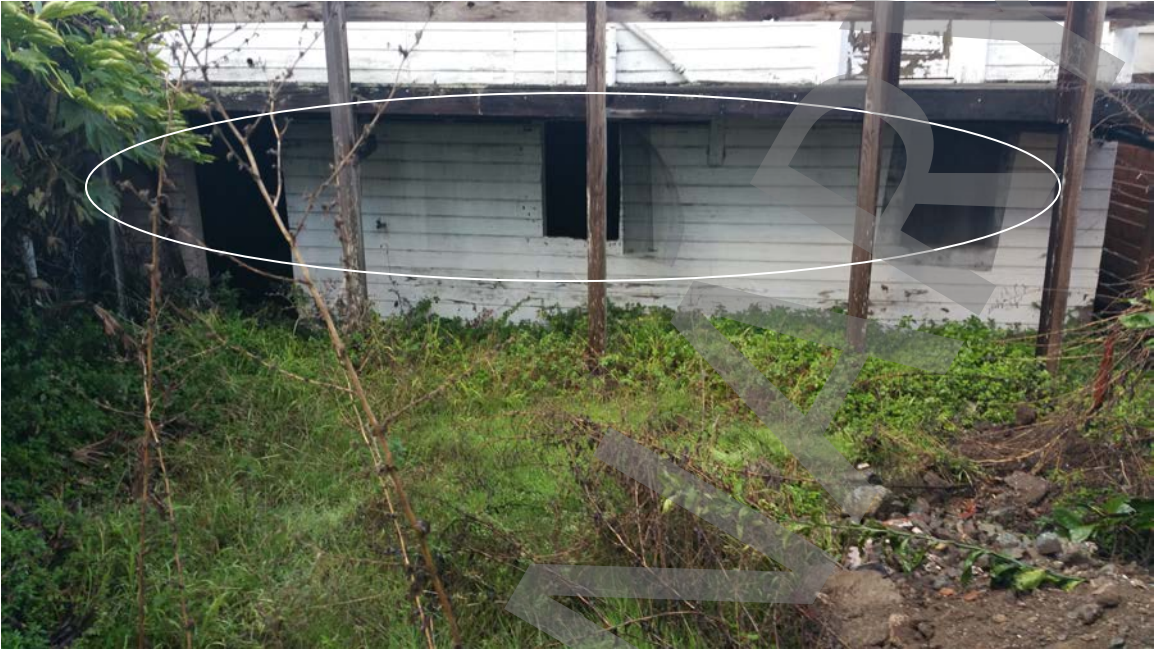
Photo # 23: Missing and broken windows and doors.
