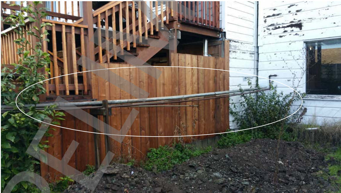
Photo # 28: Improperly placed piping. Inadequately supported, not to code.
