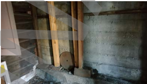
Photo # 36: Homemade, unsafe built very out of plumb posts on improper foundation, typical.
