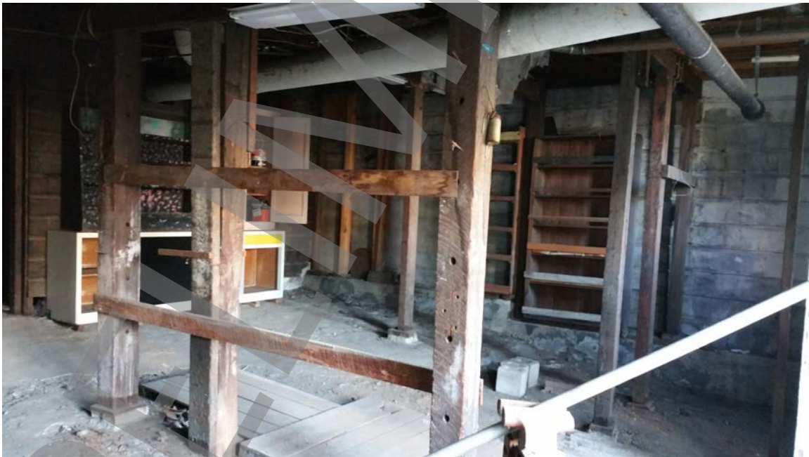
Photo # 40: Maze of homemade-design posts and beams, unable to carry required loads, throughout. Undersized joists and beams, throughout.
