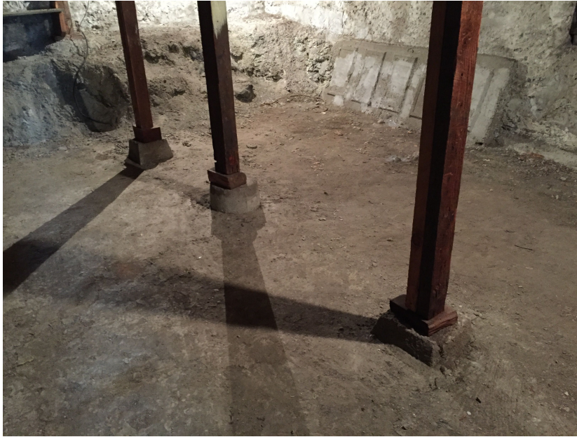
Photo 25: This photo shows the footings for the posts supporting the central beam in the original building. Note the haphazard blocks; the center post aligned at the edge of the barrel footing; and the impression of a door at the base of the retaining wall beyond. The latter feature is likely a result of using the door as a form to place concrete as infill where the footing was undermined when the area was excavated to create more usable storage space.
