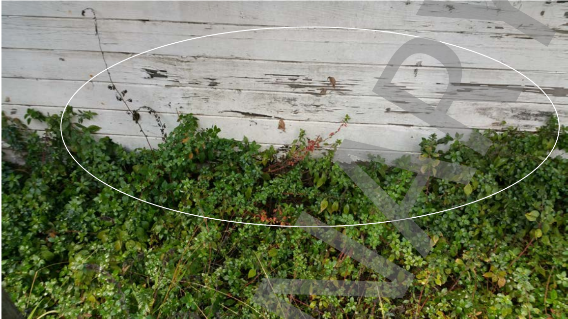
Photo # 25: Rotten siding causing peeling lead paint.
