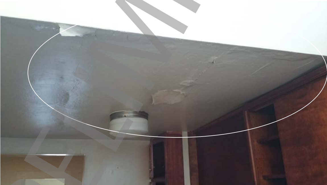
Photo # 9: Water damage to ceiling and electrical fixtures.
