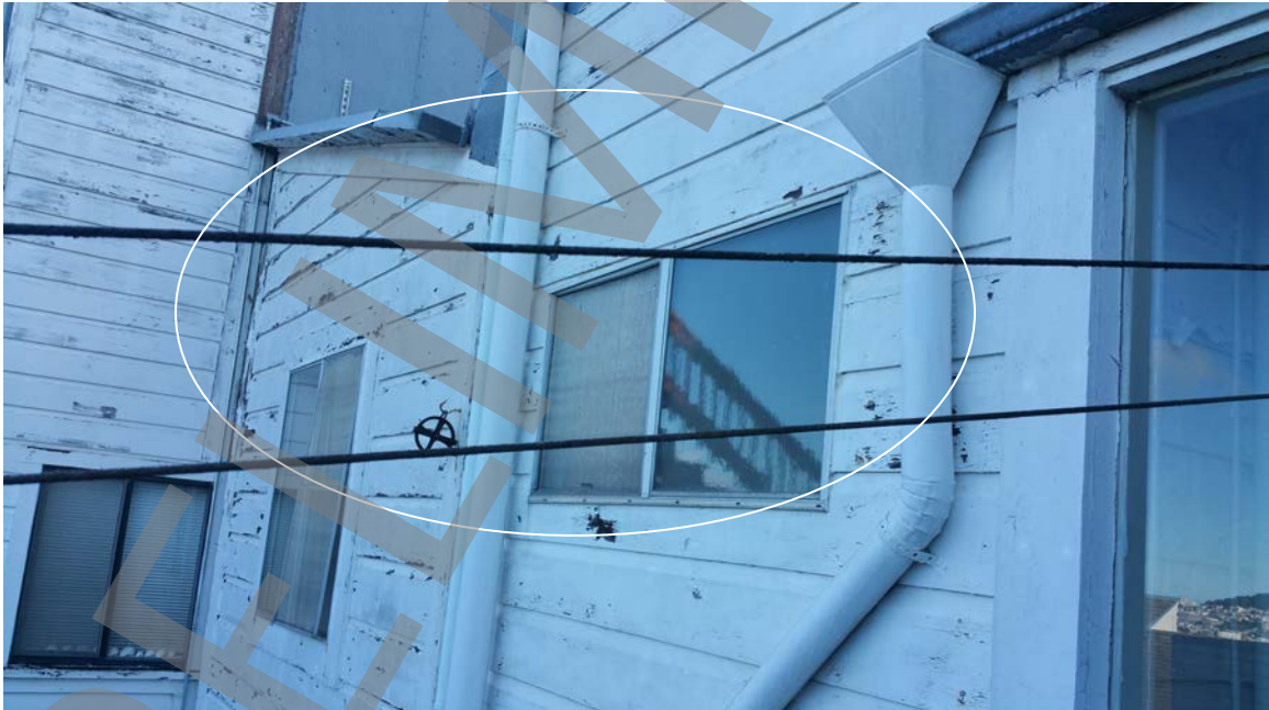
Photo # 14: Improper flashing, improper waterproofing detailing, rot, peeling lead paint at the back of the house.
