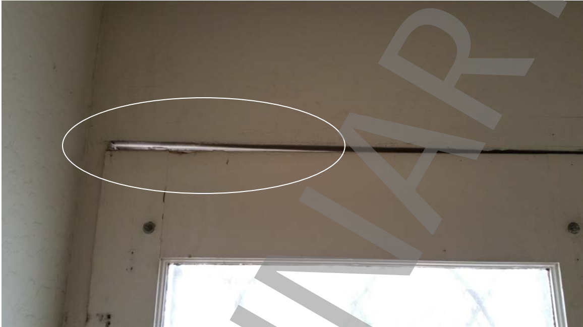
Photo # 41: The structure is uneven and moving.
