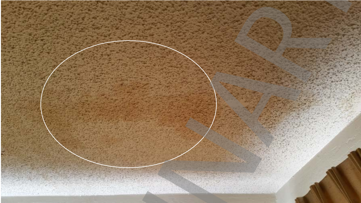
Photo # 4: Asbestos ceiling finish in living room and dining room.
