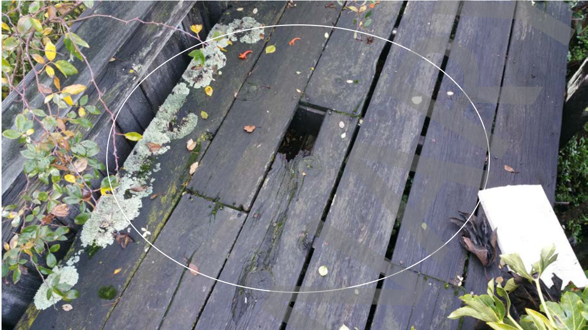
Photo # 16: Rotten, broken, elevated walkway in dangerous condition. No fire-wall, improper and unsafe railing, dangerous to all and to children especially.
