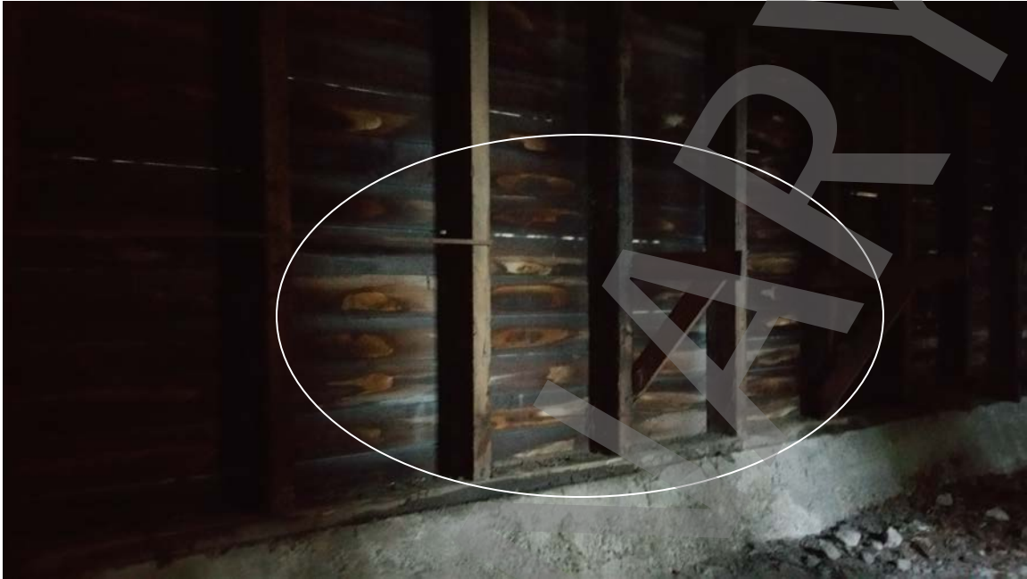
Photo # 27: Back structure water damaged, infested with pests; beetles, termites, rot.
