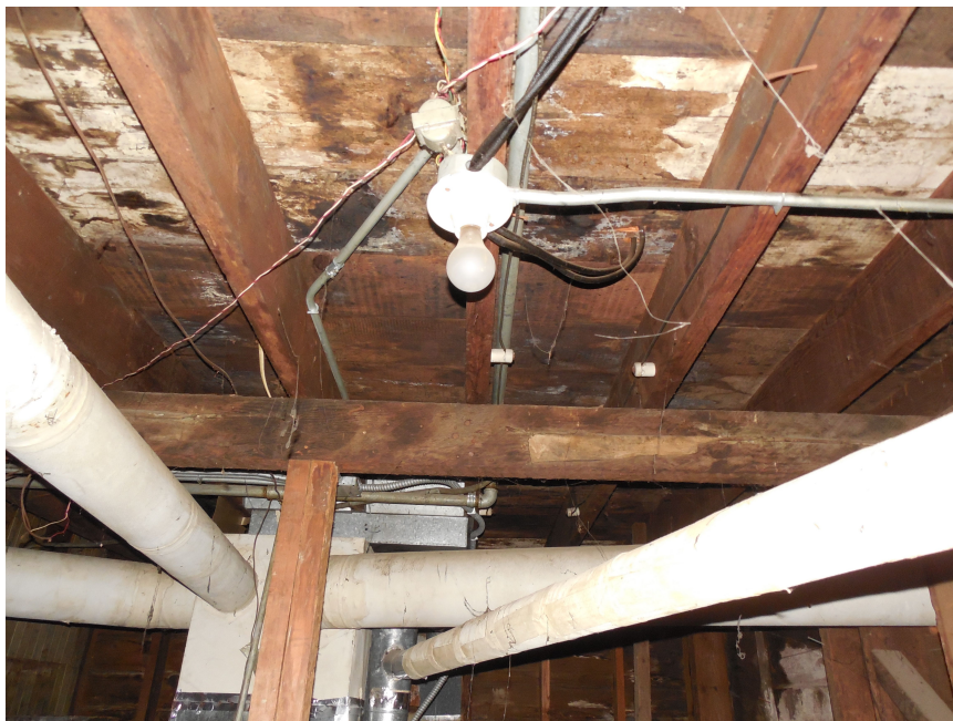
Photo 26: This photo documents the asbestos insulation for the heat ducts. The furnace is located in the small storage room under the original structure.
