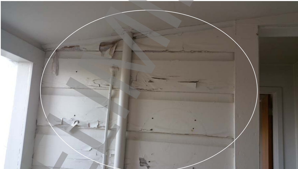
Photo # 12: Flaking and peeling asbestos finish in dining room.
