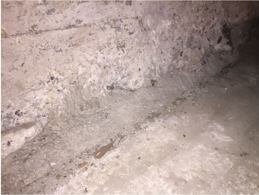
Photos 9 & 10: These photos show the base of the north perimeter footing. Note that the foundation on this side of the building has also been undermined, and a small thin patch of concrete has been added at the base of the wall to cover the exposed soil where the bottom of the footing was exposed.
