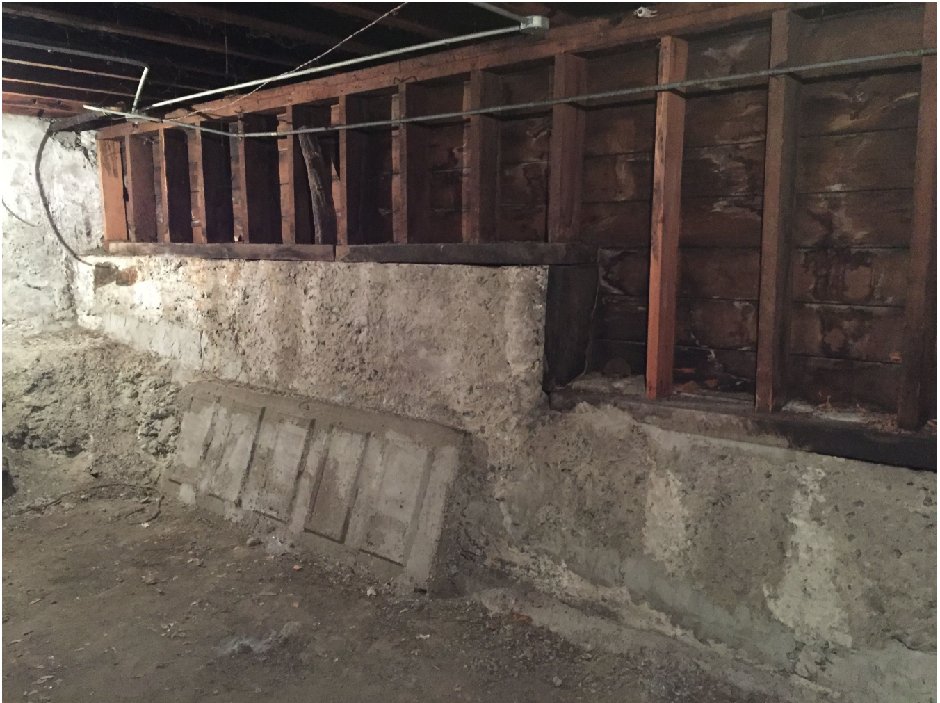
Photo 1: This photo shows the condition of the retaining wall along gridline D and the corner with the front property line retaining wall along gridline 1 (left side of photo). There are several things that indicate that the original walls were over-excavated. First, the most obvious is the patch located at the bottom of the taller portion of the wall towards the front of the building. Clearly, the wall steps down above grade, and the assumption is that it stepped down at the bottom of the wall as well. When the excavation was extended past that below-grade step, it undermined the base of the retaining wall. A patch was then made to cover the exposed soil below the bottom of the footing, and formed using a door. Although inadequate, this patch was an attempt to ameliorate the deficiency caused by excavating below the bottom of the original retaining wall. The second clue is the presence of multiple places where newer concrete has been troweled over patches of the original concrete at the base of the wall. Most likely, these areas were originally below grade, and they included rough surfaces from the side of the original excavation that formed the trench for the base of the wall, and possibly voids in the concrete. Once exposed by additional excavation, they were then patched to cover the defect. Finally, the third clue is the presence of a thin triangular fill at the base of the shorter portion of the wall (at the lower right corner of the photo). This suggests that, similar to the large door patch, the bottom of the original retaining wall was exposed and patched.
