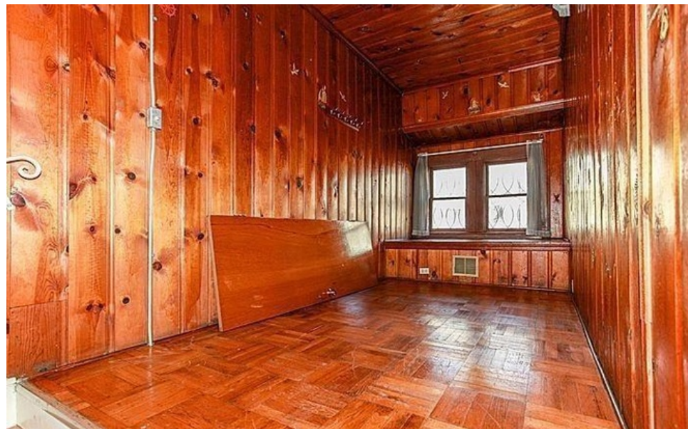
Photo 6: This photo shows the room over the driveway. This room is elevated above the rest of the floor area because it was created by filling in the area over the driveway at a level that would have still allowed a car to access the space below.
