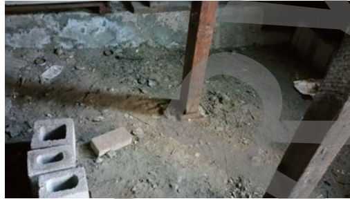
Photo # 35: Improper wood separation in area without weather protection, beetle infestation, rot.
