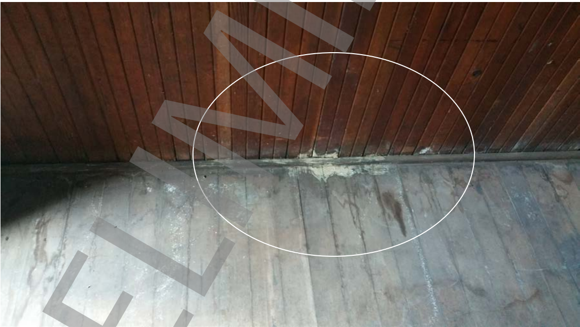
Photo # 20: Fungus and water damage at back structure: leaking walls.
