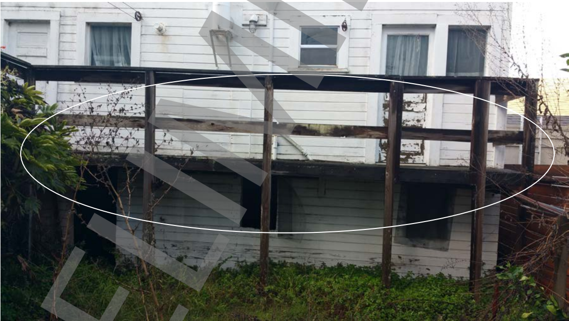
Photo # 24: Rotten walkway and peeling lead paint.
