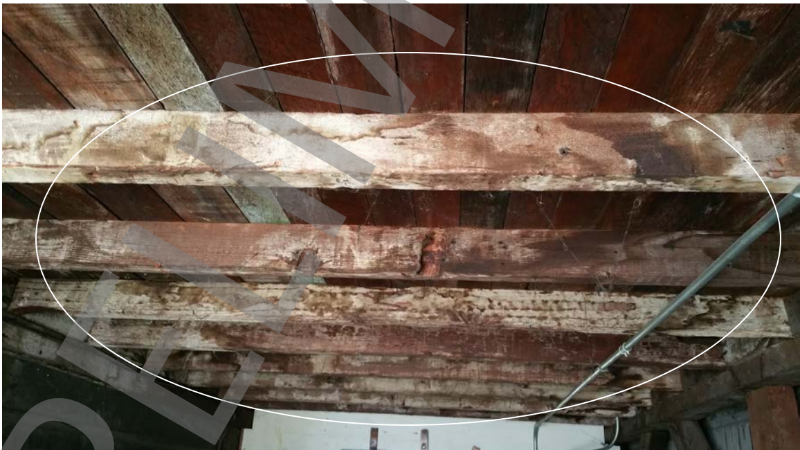
Photo # 42: Undersized floor joists, typical.
