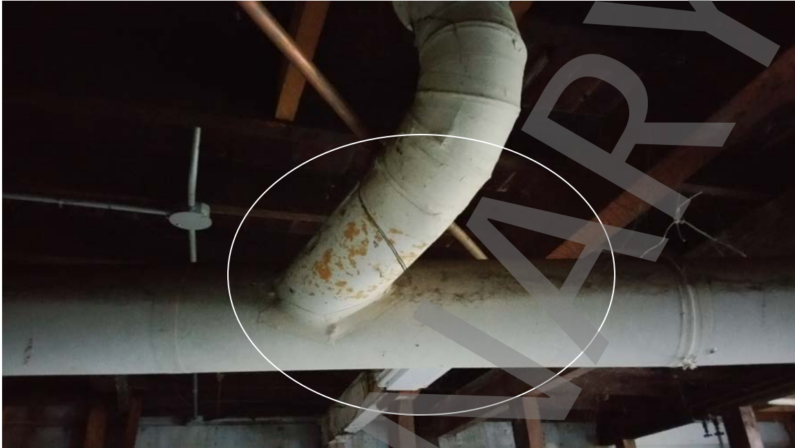
Photo # 33: Asbestos piping must be removed to replace the substandard joists and subfloor.
