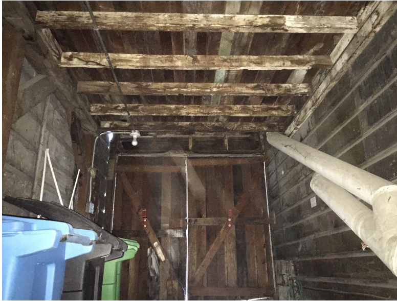
Photo 13: This photo shows the infill section at the north of the original structure. The floor framing supports the unconventional elevated room adjacent to the living room. Note that the framing is supported at the property line by post and beam construction—not a studwall—and that the siding for the adjacent building can clearly be seen. This condition leaves no separation between the two adjacent properties.
