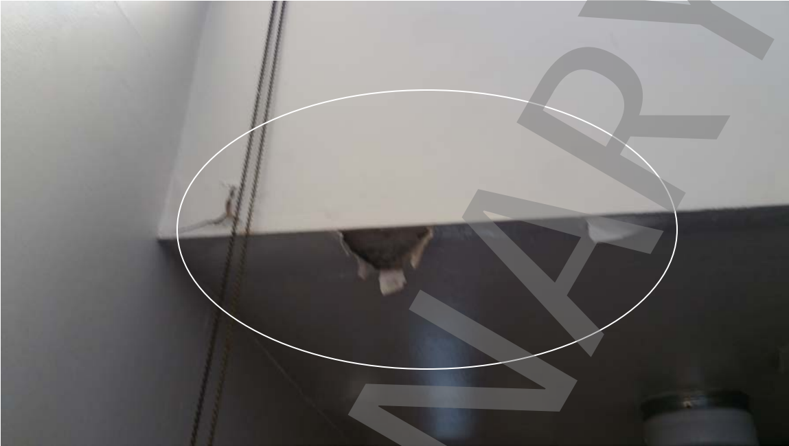
Photo # 8: Water damage to roof, wall and ceiling at kitchen.
