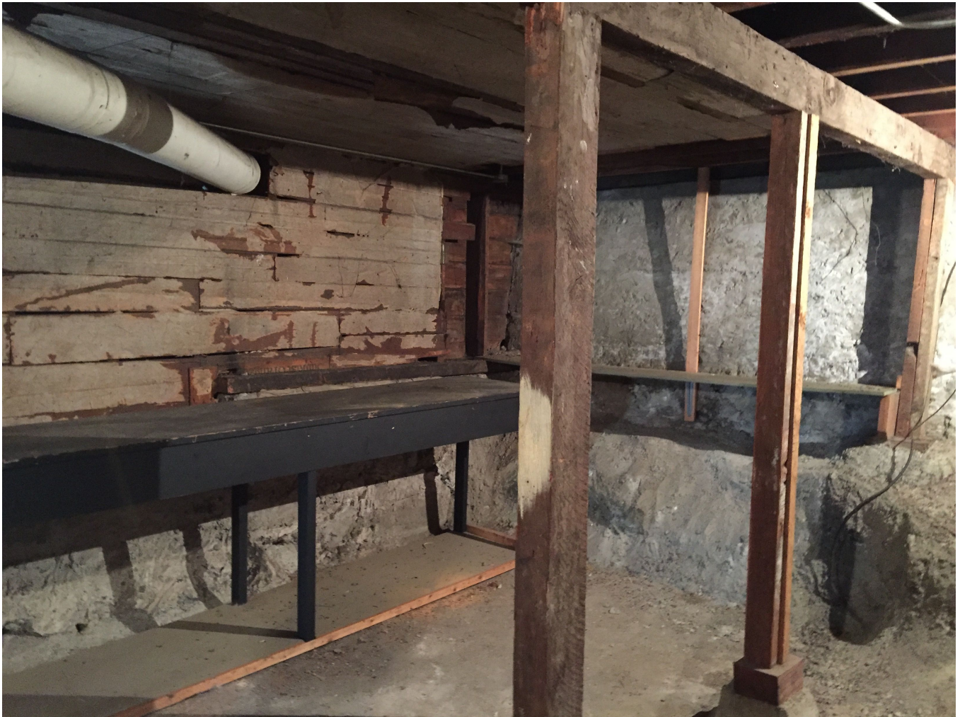
Photo 8: This photo shows the north side of the perimeter foundation for the original building along gridline B. This was probably a short retaining wall like the one on the south side that has been so badly undermined, but the addition of the carriage house and the access driveway along the north side of the property probably eliminated the retained portion of soil on the other side of this wall. Consequently, this is no longer a retaining wall, and it now just functions as a typical spread footing. Nonetheless, this wall has been undermined in a similar way to the one across from it.
