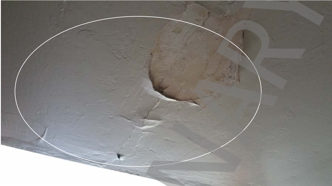
Photo # 10: Water damage to ceiling from leaking roof.
