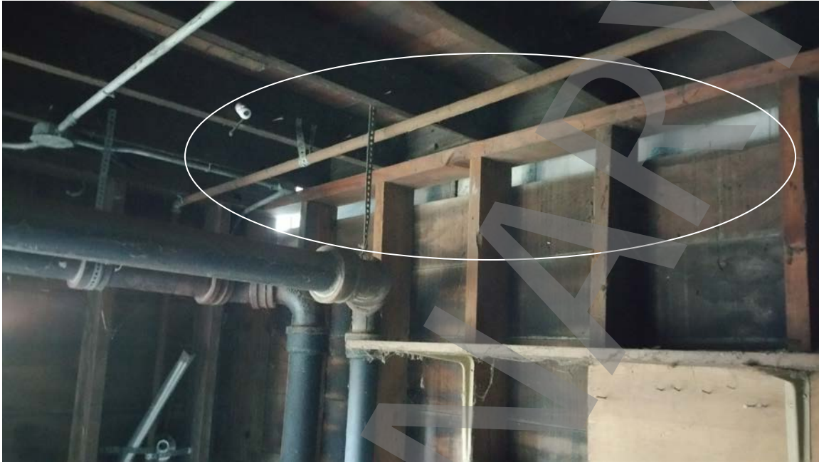
Photo # 31: Holes in the side walls of the building, typical. No shear protection against earthquake motion.
