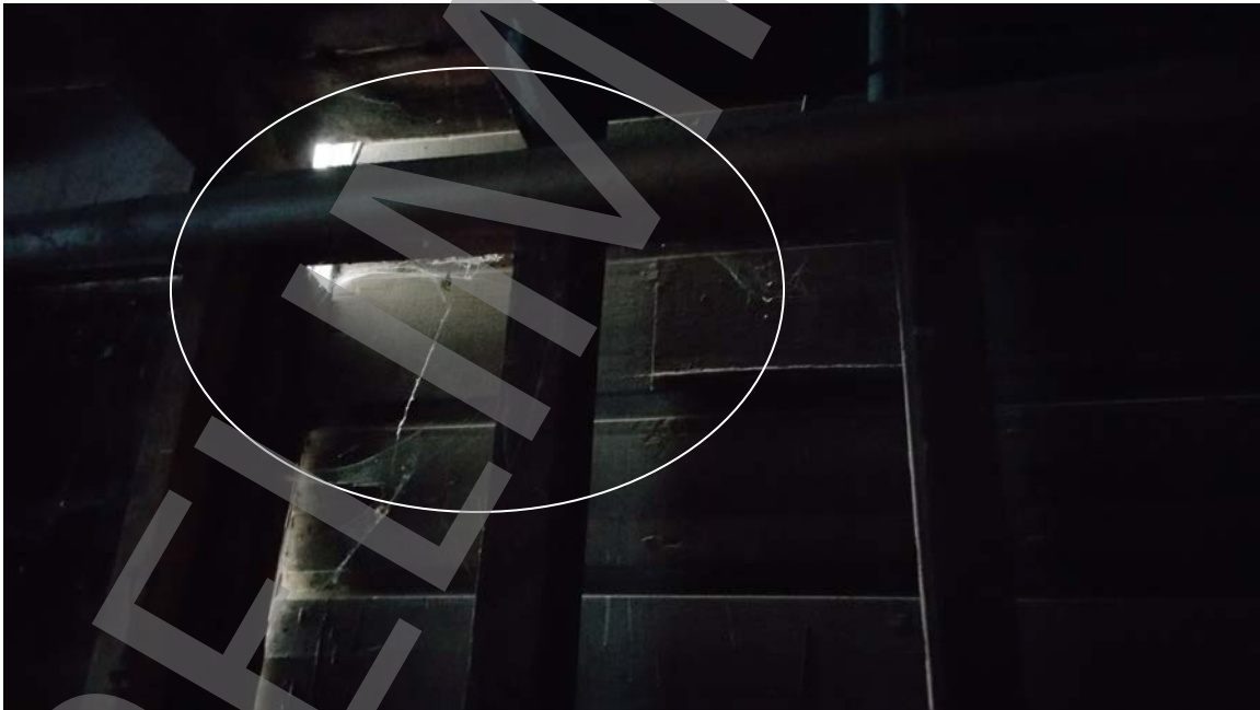
Photo # 31: Holes in the side walls of the building, typical. No shear protection against earthquake motion.
