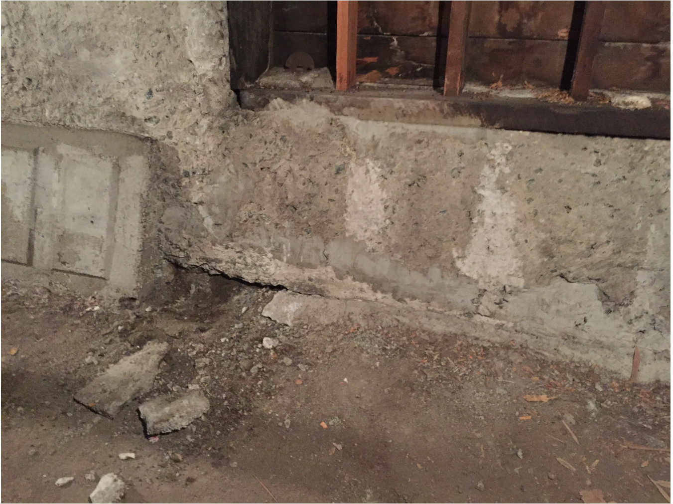
Photo 5: This photo shows the area adjacent to the large patch, where a thin patch was placed along the bottom edge of the shorter retaining wall section. We removed a section of this smaller patch, which exposed the bottom of the original retaining wall. Like the larger patch, this indicates that the secondary excavation went below this section of the original footing as well. This photo also shows some of the areas where new concrete has been skimmed over what are presumably voids in the original concrete. Notice how these skim patches follow a gradual upward line from right to left. To me, this suggests that that was the original grade level, which sloped up towards the front of the building.
