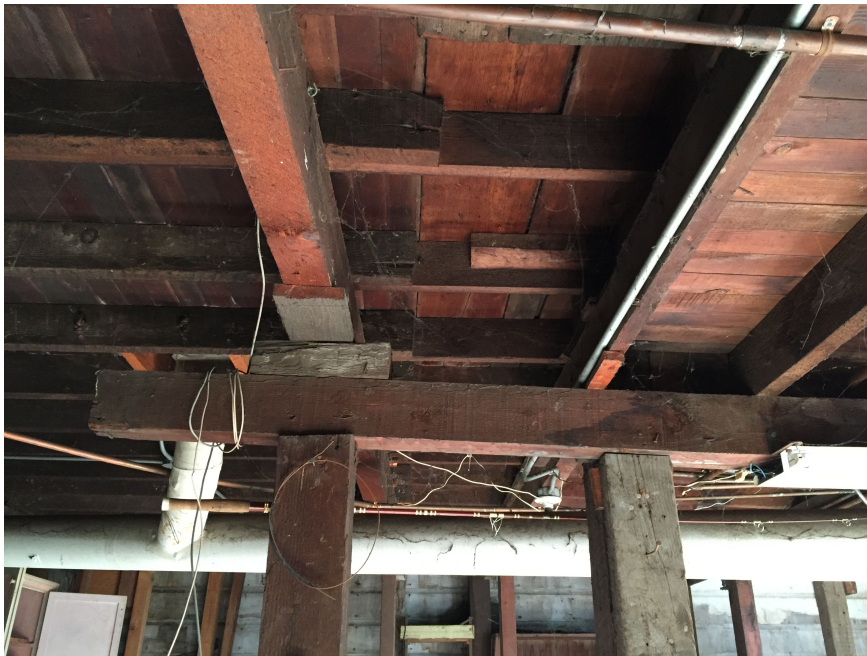
Photo 17: This photo shows the floor framing above the north property line at the rear from the previous photo. Note the three distinct sections of floor framing—left, middle, and right—along with changes in framing direction. The beam is at gridline 7. The framing at the left is somewhat mysterious, because it appears that there are two levels of floor framing, one on top of the other. The area corresponds to Bedroom 3, and there is no change in elevation between the Dining Room and Bedroom 3.
