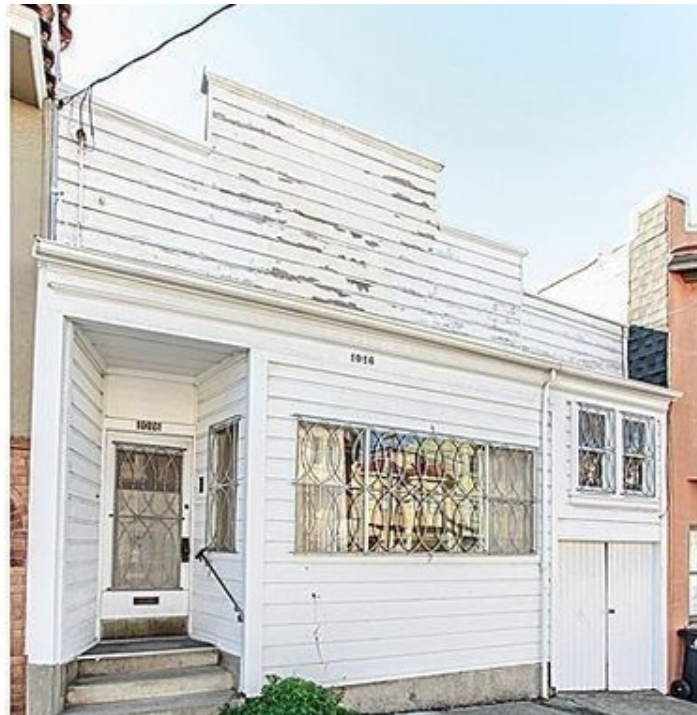
Photo 11: Note the false façade, and the extension to the right (north) over the garage doors. The three sections of this element are symmetrical over the original structure, but the section to the right does not match, indicating that it was added later. A vertical joint can also be seen at the interface between the new and old sections. Also note the extension of the front of the building, projecting forward of the false façade above. This was likely part of the 1924 permit.
