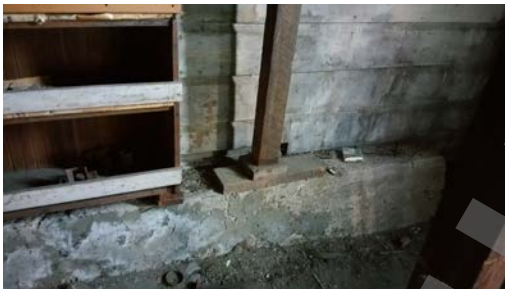
Photo # 36: Homemade, unsafe built very out of plumb posts on improper foundation, typical.
