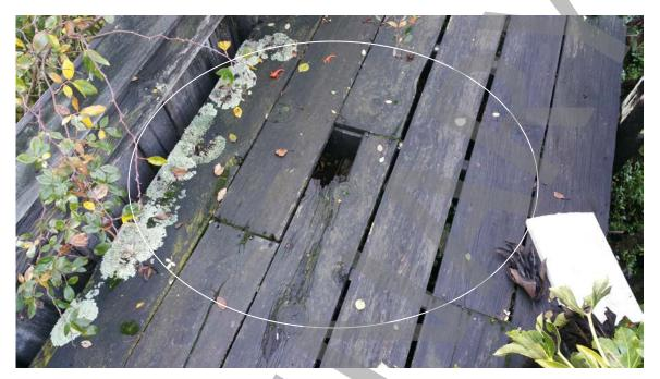
Photo # 16: Rotten, broken, elevated walkway in dangerous condition. No firewall, improper and unsafe railing, dangerous to all and to children especially.
