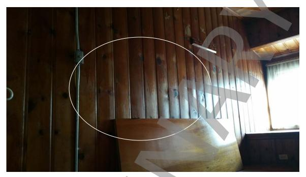
Photo # 6: Property line wall not fire resistant. Inadequate floor joists throughout.
