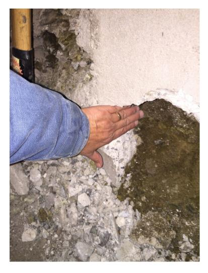
Photos 3 & 4: In these photos I use my hand as a reference to demonstrate the depth of the door patch. Note that the depth of the patch is roughly the depth of my fingers at the top of the patch, and also that it is the same depth below where the soil is exposed. This indicates that the original retaining wall did not extend down to the bottom of the current floor level, and that it was undermined with the secondary excavation.
