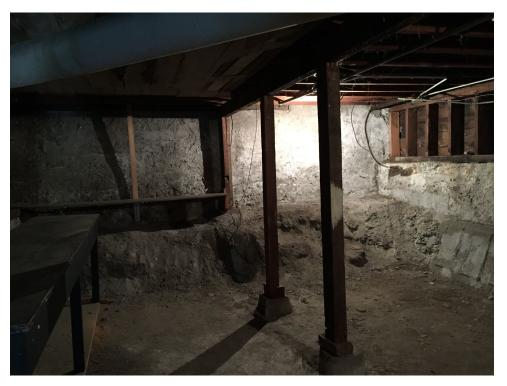
Photo 6. This photo shows the retaining wall at the front property line. Note that the original wall only extends down about 1/2 to 2/3 of the current total headroom depth. The bottom portion is crudely excavated and covered with rat slab, and provides no confinement or support of the base of the original retaining wall.
