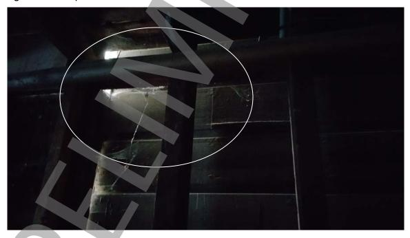
Photo # 32: Holes in the building, typical. Building is not waterproof.
