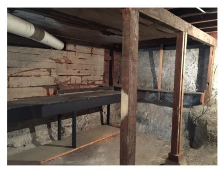
Photo 24: This photo shows the central post and beam system at the original section of the building. The narrow building, combined with the central support renders the floor joists adequate, but the beam does not meet the demand imposed by the loads required by the code in effect at the time of original construction. This beam needs to be replaced.
