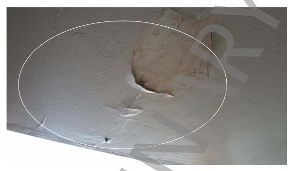
Photo # 10: Water damage to ceiling from leaking roof.
