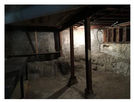
Photo 10: This photo shows the basement area under the original building. Note the retaining wall at the back, which has been undermined in order to create more headroom at the rear of the storage area.
