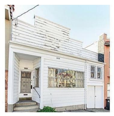
Photo 11: Note the false façade, and the extension to the right (north) over the garage doors. The three sections of this element are symmetrical over the original structure, but the section to the right does not match, indicating that it was added later. A vertical joint can also be seen at the interface between the new and old sections. Also note the extension of the front of the building, projecting forward of the false façade above. This was likely part of the 1924 permit.
