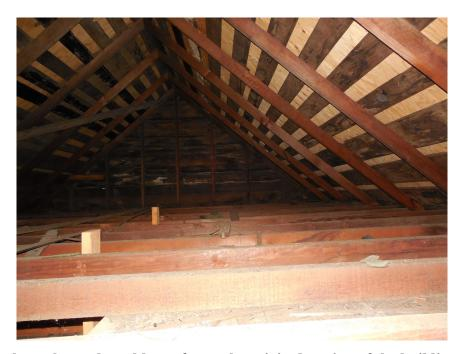
Photo 22: This photo shows the gable roof over the original section of the building. Note the long spans on the rafters, with no collar ties or kickers. Note also the 2x4 stickers hanging down to support the dropped ceiling below.
