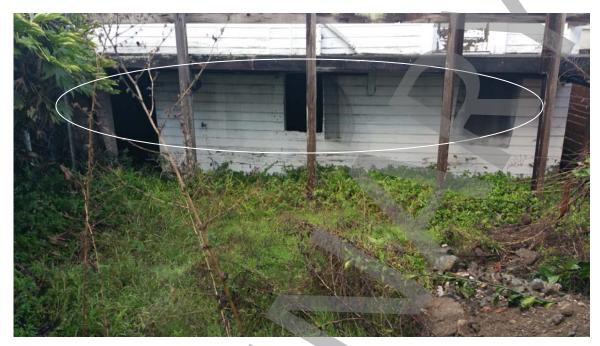
Photo # 23: Missing and broken windows and doors.
