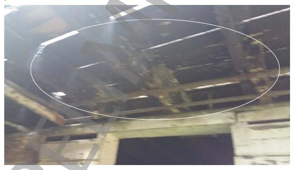
Photo # 26: Rotten framing and missing siding and waterproofing.
