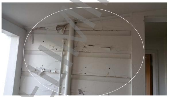
Photo # 13: Excessive moisture, rot, leaking, at mud room.
