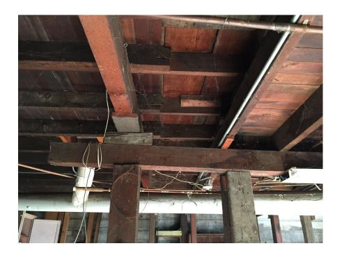
Photo 18: This photo shows a section of the central longitudinal beam at in the rear addition area. Note the three distinct floor framing sections of different depth. The use of shims to support the crossing beam is completely unorthodox for any period of construction, and highlights the piecemeal approach to the building's expansion.
