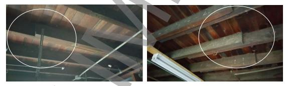
Photo # 34: Undersized joists, and spliced at mid-span, typical!
