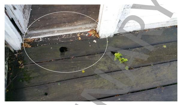
Photo # 19: Peeling lead paint and chips at back structure.
