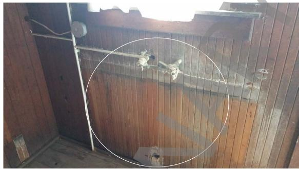
Photo # 21: Missing sink and drain.
