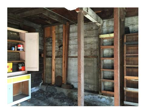
Photo 20: this photo shows the area to the left of the previous photo. Note the funky posts, propped up on blocks, supporting the corner of the addition. Again, this is a completely unorthodox method of construction.
