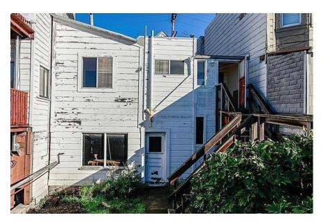
Photo 12: This photo shows the rear of the building, where three distinct roof sections are clearly visible beyond the original gable. This corresponds with the roof plan shown on sheet A-103.
