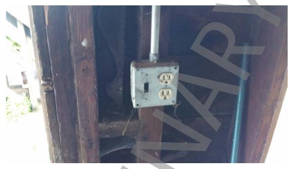
Photo # 39: Broken and improperly installed electrical throughout.
