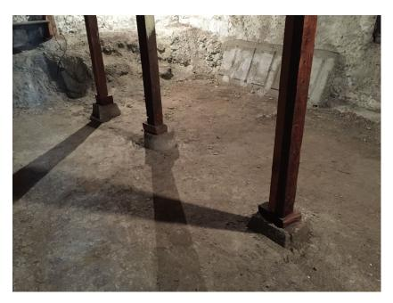
Photo 25: This photo shows the footings for the posts supporting the central beam in the original building. Note the haphazard blocks; the center post aligned at the edge of the barrel footing; and the impression of a door at the base of the retaining wall beyond. The latter feature is likely a result of using the door as a form to place concrete as infill where the footing was undermined when the area was excavated to create more usable storage space.
