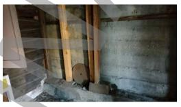
Photo # 36: Homemade, unsafe built very out of plumb posts on improper foundation, typical.
