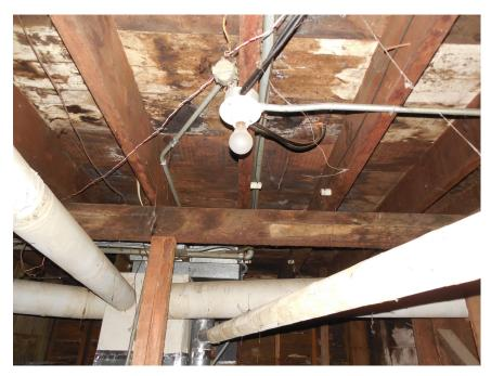
Photo 26: This photo documents the asbestos insulation for the heat ducts. The furnace is located in the small storage room under the original structure.
