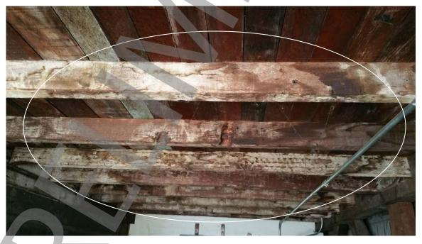
Photo # 42: Undersized floor joists, typical.
