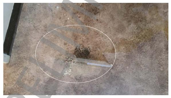
Photo #7: Water leaking onto kitchen floor from roof and skylight.
