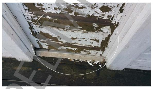
Photo # 17: Rotten door with peeling lead paint, and chips on the ground, at main house back door.
