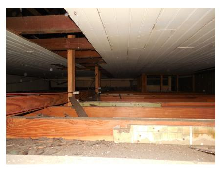
Photo 23: This photo shows the interstitial space between the original ceiling, clad in T&G beadboard, and the dropped ceiling.
