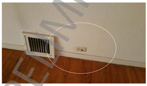
Photo # 11: Broken and improperly placed electrical outlets, and other fixtures.
