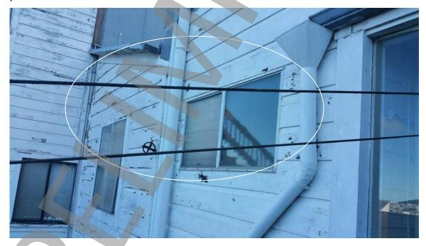
Photo # 15: Improper waterproofing and flashing. No trim.
