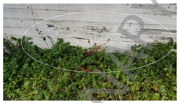
Photo # 25: Rotten siding causing peeling lead paint.
