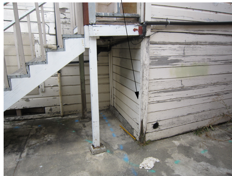
Foundation Detail - Wood in contact with grade; decay
