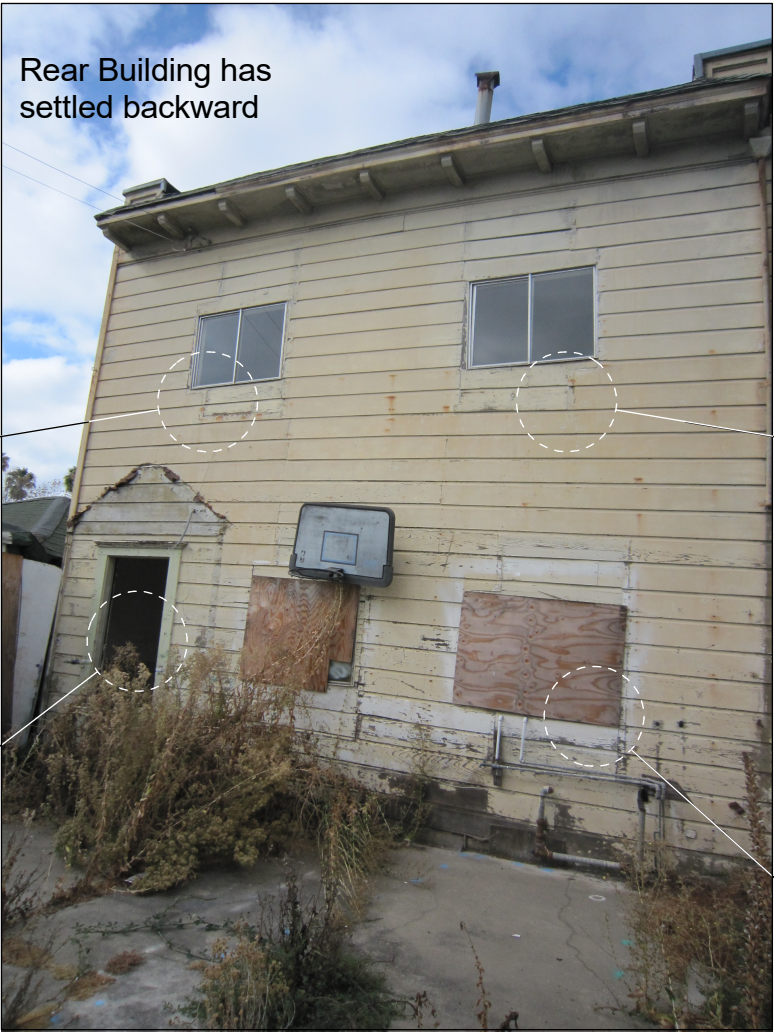
Entire Building has fallen backward off rear foundation
