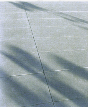
Required saw-cut joints
