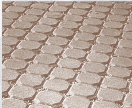
Required saw-cut joints
