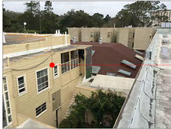
2-STORY BUILDING WEST ON STANYAN
