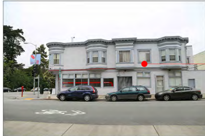
2-STORY BUILDING WEST ON STANYAN
