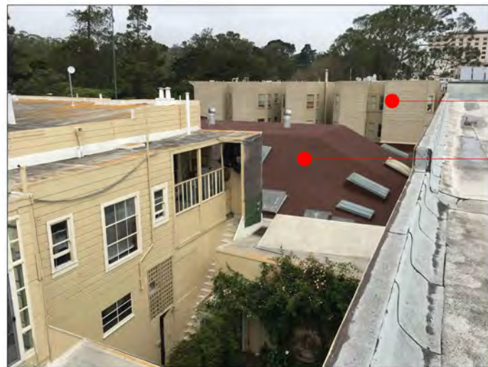
BUILDINGS NORTHWEST ON STANYAN & OAK
