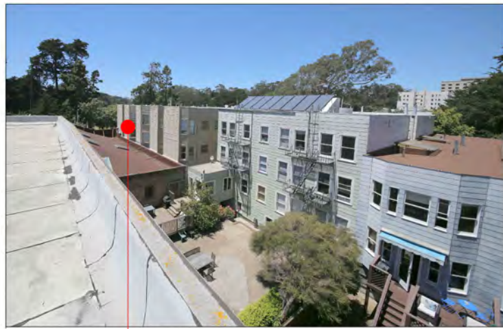
LOOKING TOWARDS NORTHWEST, 4-STORY HIGH BUILDING
