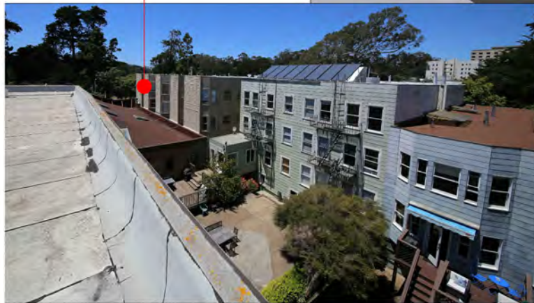
BUILDINGS NORTHWEST ON STANYAN & OAK
