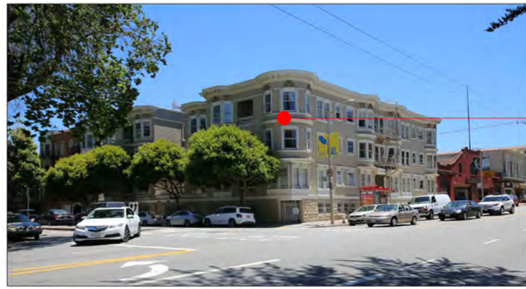
BUILDINGS NORTHWEST ON STANYAN & OAK
