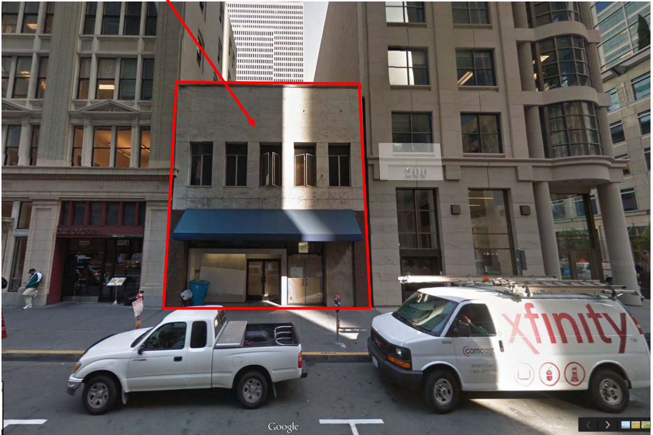
Street View of 212-214 California Street (view from California Street)
