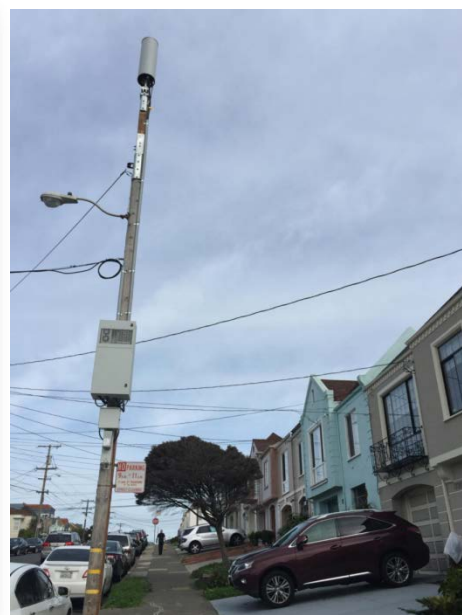
Crown Castle, for Verizon Wireless “oDAS XL” Personal Wireless Services Facilities, in the Outer Sunset. The bulky nature and potential noise generation from cooling fans on residential streets is disfavored.
