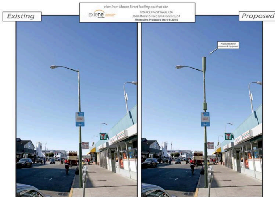
Extenet Systems, for Verizon Wireless “oDAS R” (or Small Cell) on a steel light pole owned by the City (SF Public Utilities Commission). An antenna is located on top and two computers (equipment) are located midway down the pole. Planning Department staff worked with the Department of Public Works, and the carrier to create a bracket to “screen” one of the computers with road signage.
