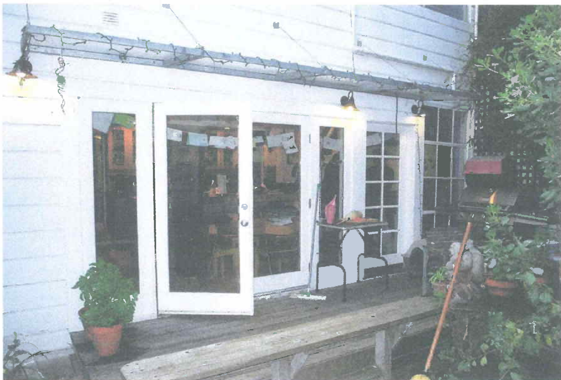
Details of windows and doors in the east side of the house. The former are original or early, while the latter appear to be of recent construction.
