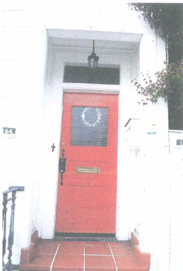
Above and at right: Entrance of house, with details showing paneled sides, transom, and front steps.
