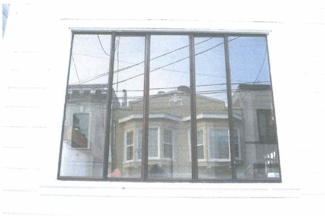
Window in the main facade. The metal sash is an alteration. The opening with its plain board trim and sill may be original, but this is uncertain.
