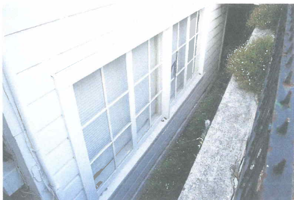
Window in the main facade. The metal sash is an alteration. The opening with its plain board trim and sill may be original, but this is uncertain.
