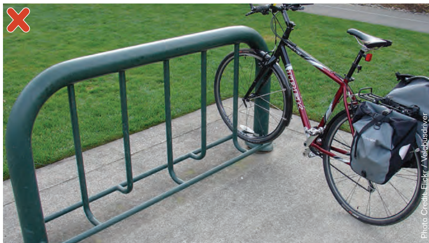
Rack design does not allow for bicycles to be properly secured
