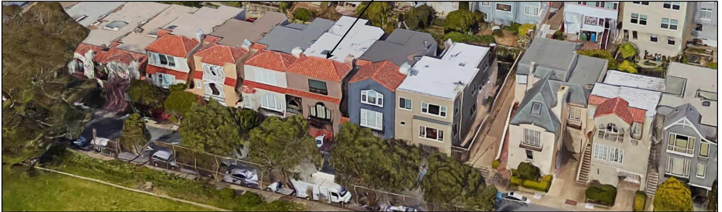
ROSSI AVENUE STREET FACADES ON BOTH SIDES OF SUBJECT PROPERTY
