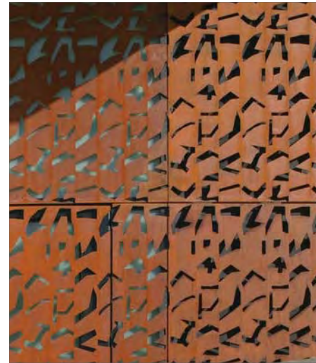
11 ORNAMENTAL PANEL / FENCE / GUARDRAIL SYSTEM, TYP. (WEATHERING STEEL PREFERRED)
