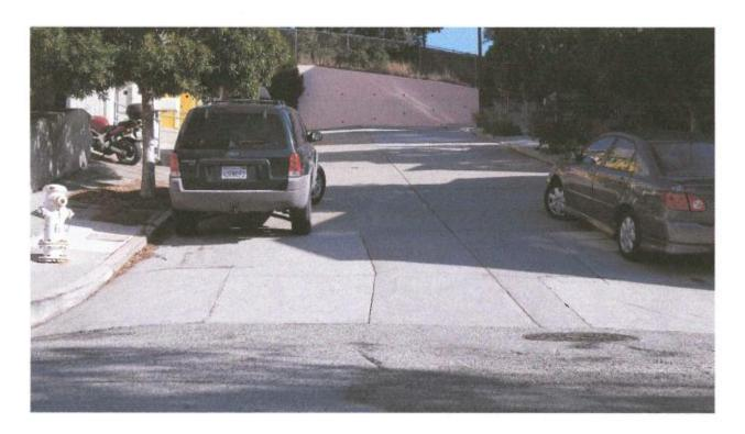
This is the next street, Banks St, and shows how a retaining wall is necessary to reduce the grade and allow proper road access for residential dwellings. This is not possible on Folsom St.
