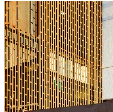
Corten screen with custom cut-out pattern at West Stair. Cut-out Pattern TBD.
