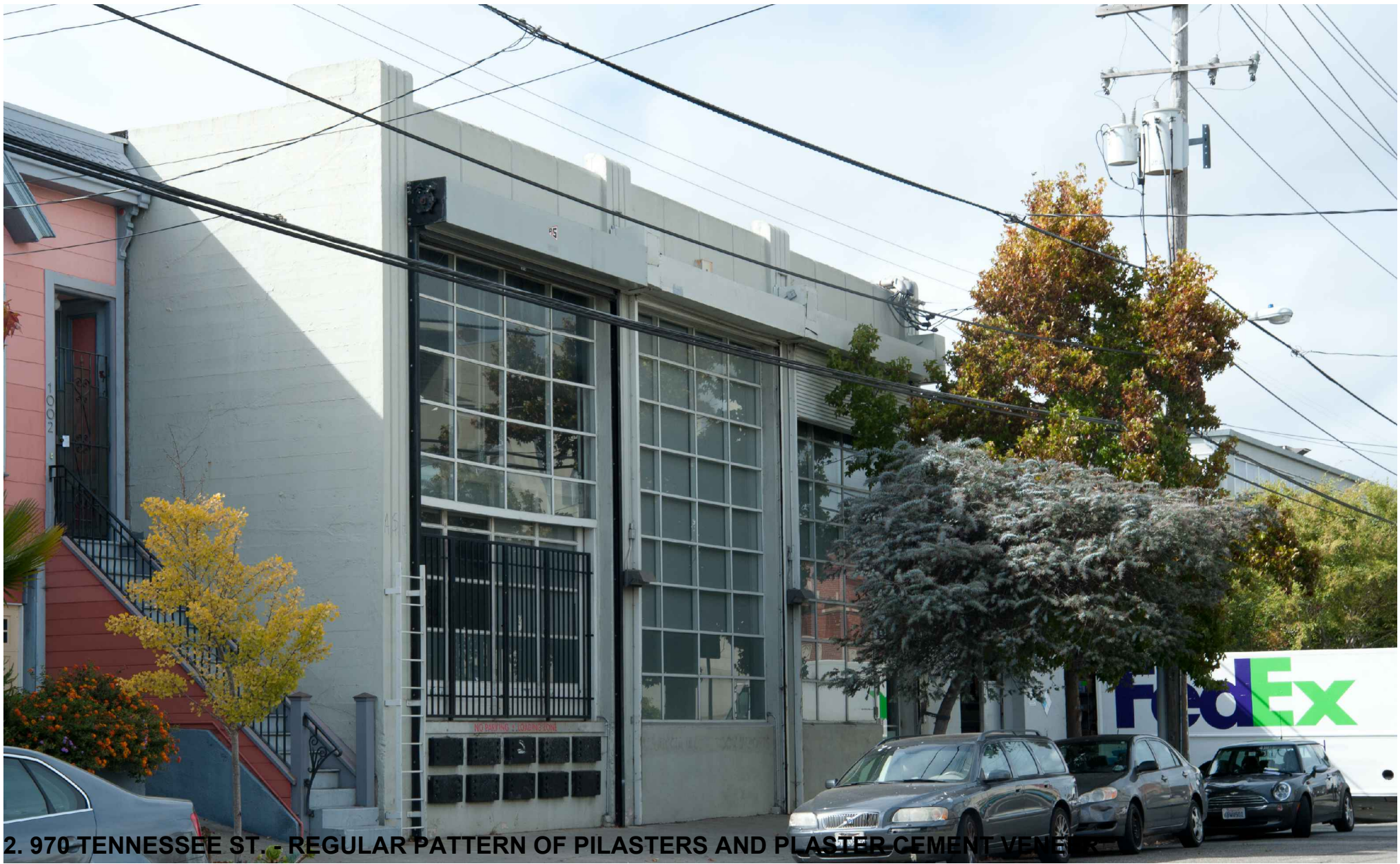
2. 970 TENNESSEE ST. - REGULAR PATTERN OF PILASTERS AND PLASTER CEMENT VENEER
