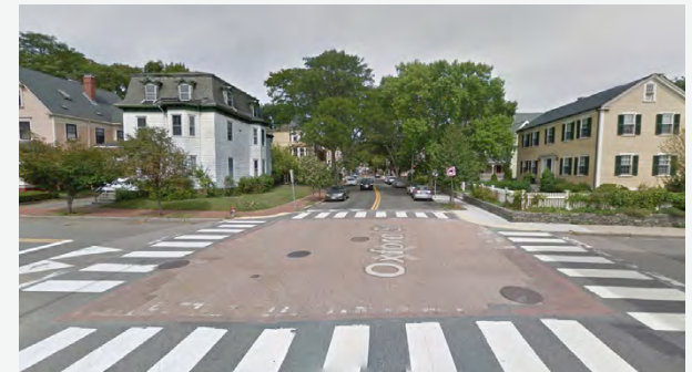
An example of a raised intersection with decorative treatment and delineated crosswalks.
