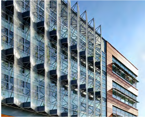
Rainscreens are decorative yet functional features. PHOTO: PERKINS+WILL
