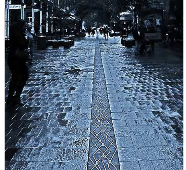
A special trench drain delineates uses or zones within a single field of paving. SOURCE: NEWTOWN GRAFFITI / FLICKR
