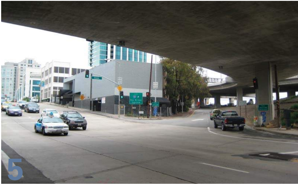
5 BELOW I-80 OFF-RAMP
