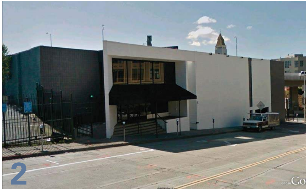
2 EXISTING BUILDING ON SITE
