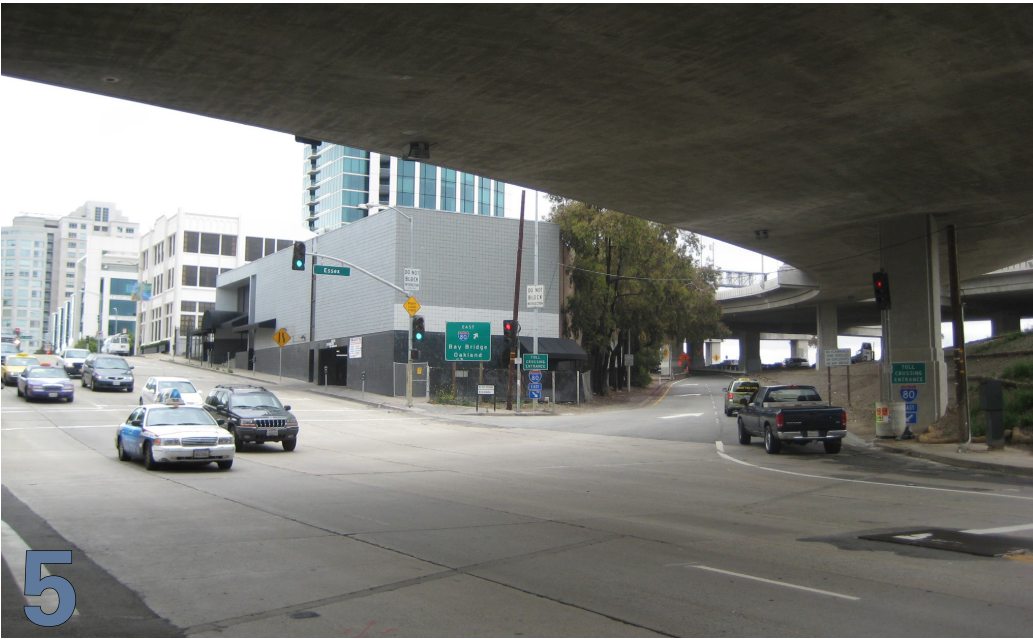
BELOW I-80 OFF-RAMP
