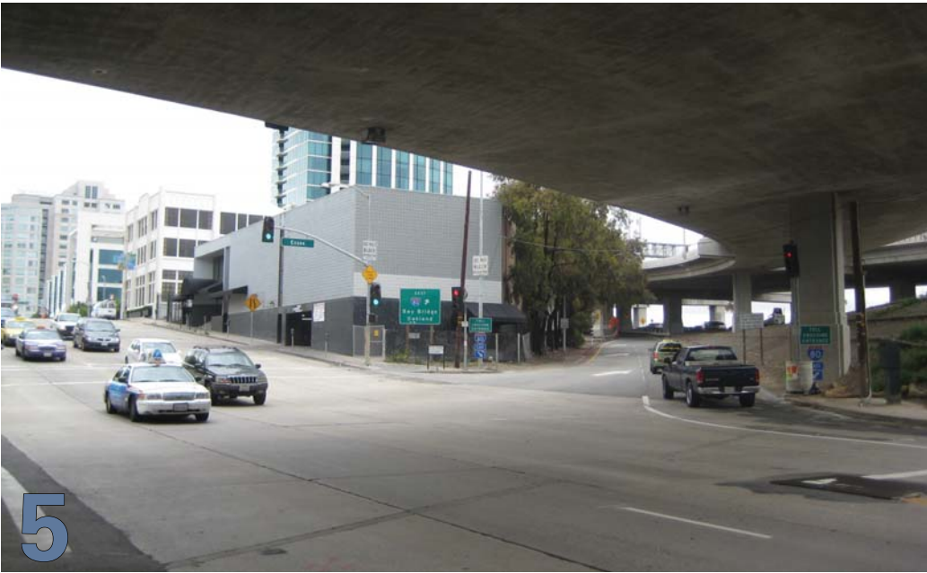
5 BELOW I-80 OFF-RAMP
