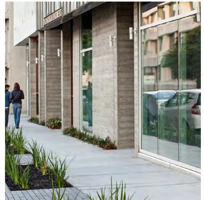
RICHARDSON APARTMENTS, DAVID BAKER ARCHITECTS BOARDFORM CONCRETE AND STOREFRONT
