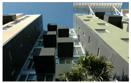
9) BALCONIES CLAD IN CLOSE MESH BAR GRATING
