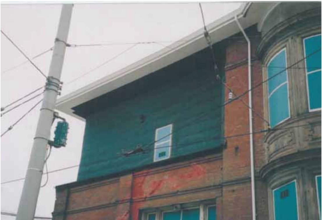
14. Office Building north elevation view of 2nd floor wall reconstruction at 1906 earthquake damage
