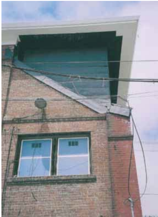
13. Office Building east elevation view of 2nd floor wall reconstruction at 1906 earthquake damage
