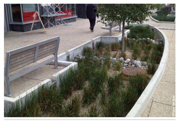
Fig. 9.4.2a Stormwater Planter
