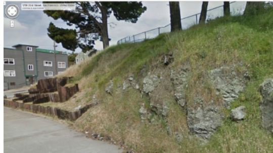
If structurally sound, cut rock should be exposed.
