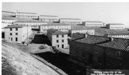
The construction of Potrero Terrace from 1941.
