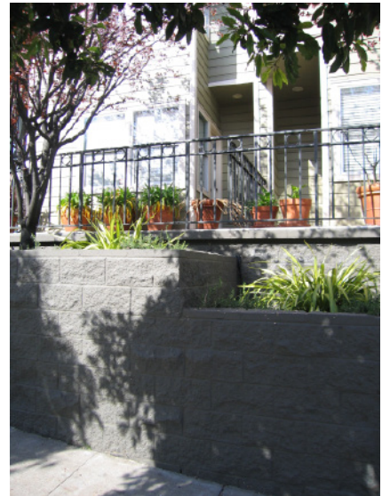
Porch area above low wall making up change in grade
