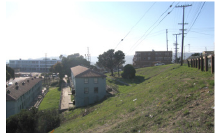
Steep slope down from 23rd Street
