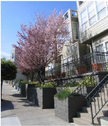
Joint porches step up steep streets
