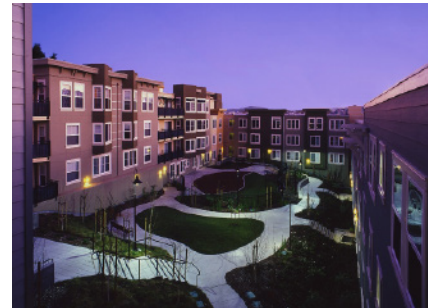
Courtyard common open space
