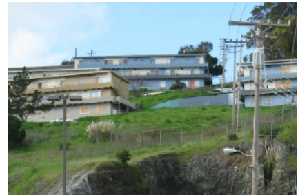
Potrero Annex above steep topography/cut
