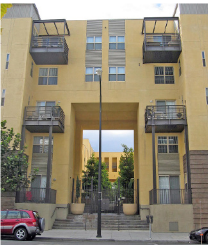
Shared portal entry
