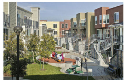
Common open space at podium level
