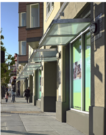
Individual awnings and columns articulate building facade rhythm.
