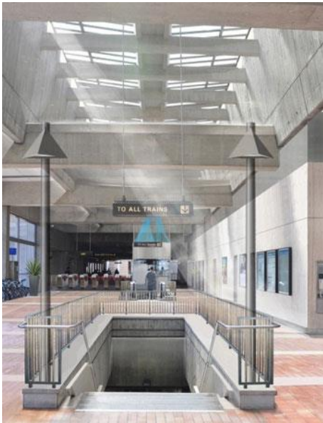
Pedestrian Improvements at Balboa Bart Station
