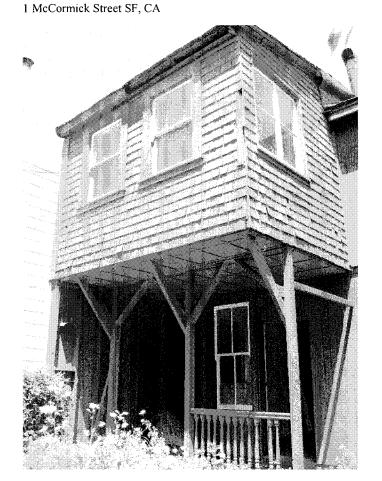
Photo 7: The rear addition was added in 1947. Its primary support is the beam and three posts seen in the photo. This addition is also the location of the worst settlement in the building—as much as 6-inches lower than the zero point at the front door. This addition is also encroaching across the property line and leaning on the adjacent building.
