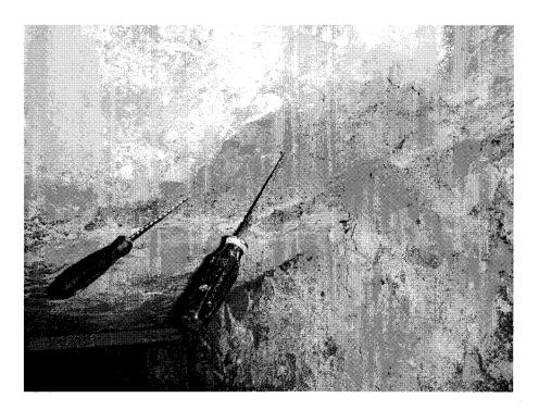
Photo 24: Section of early rubble concrete foundation. The sizable chunks of brick in the aggregate will form large voids that may not be filled with sand and cement. The likely use of beach sand further shortened the life of the concrete to the point that one can now penetrate it with a screwdriver using relatively little force.
