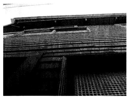
Photo 27: North elevation shows windows where the bathroom is now (note new window above the tub) that have been boarded up from the inside. Not properly filling in these openings creates a water trap.
