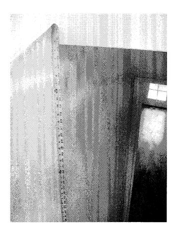
Photo 18: Clearance at stair landing between floors is only 6'-5-1/2"
