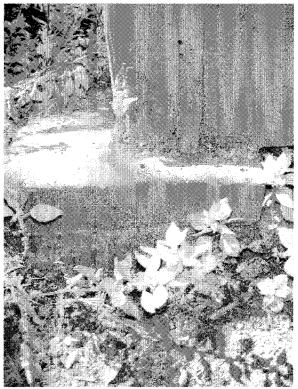
Photo 20: This is an example of improper grade, showing how an inadequate separation between the earth and wood framing members can lead to rot at the foundation interface over time.
