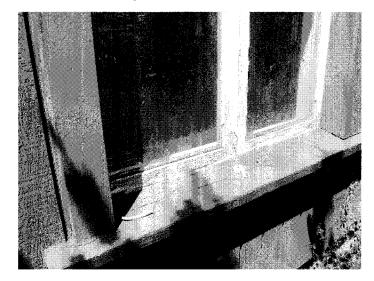
Photo 25: Typical example of exterior finishes. Note the newer T-111 siding and the failing paint, as well as the improperly installed sill that butts up against the sash, providing a path for water to enter the building.
