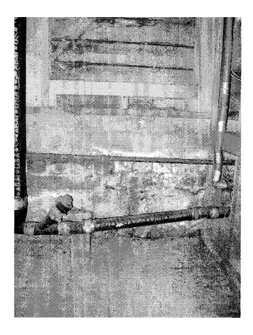
Photo 22: Section of original brick foundation augmented with concrete, presumably to address improper grade conditions.
