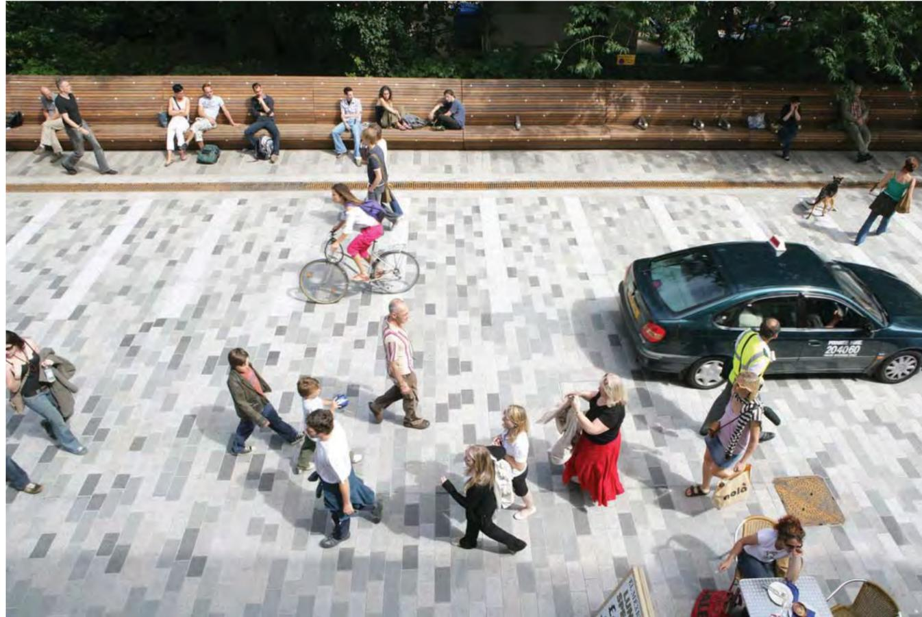
PRE-CAST UNIT PAVERS IN A GRADATION OF TONES THAT RELATE TO BOTH THE FACADE TREATMENT AND THE ADJACENT OSCAR PARK PAVING.
