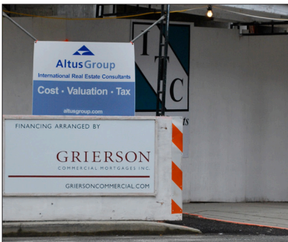
Precedent – Temporary contractor signs.
