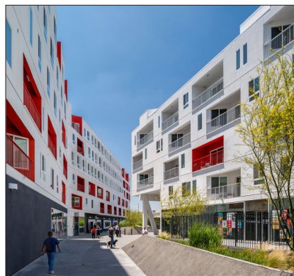
Precedent: Example of Articulation and Fenestration Strategies, such as vertical recesses, punched openings, and color variation on facade. Credits: One Santa Fe, Michael Maltzan Architecture, KTGy, Gensler, Photo © Photekt.
