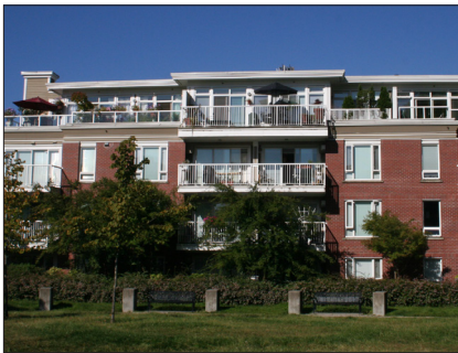
Precedent – Four to five story residential buildings.
