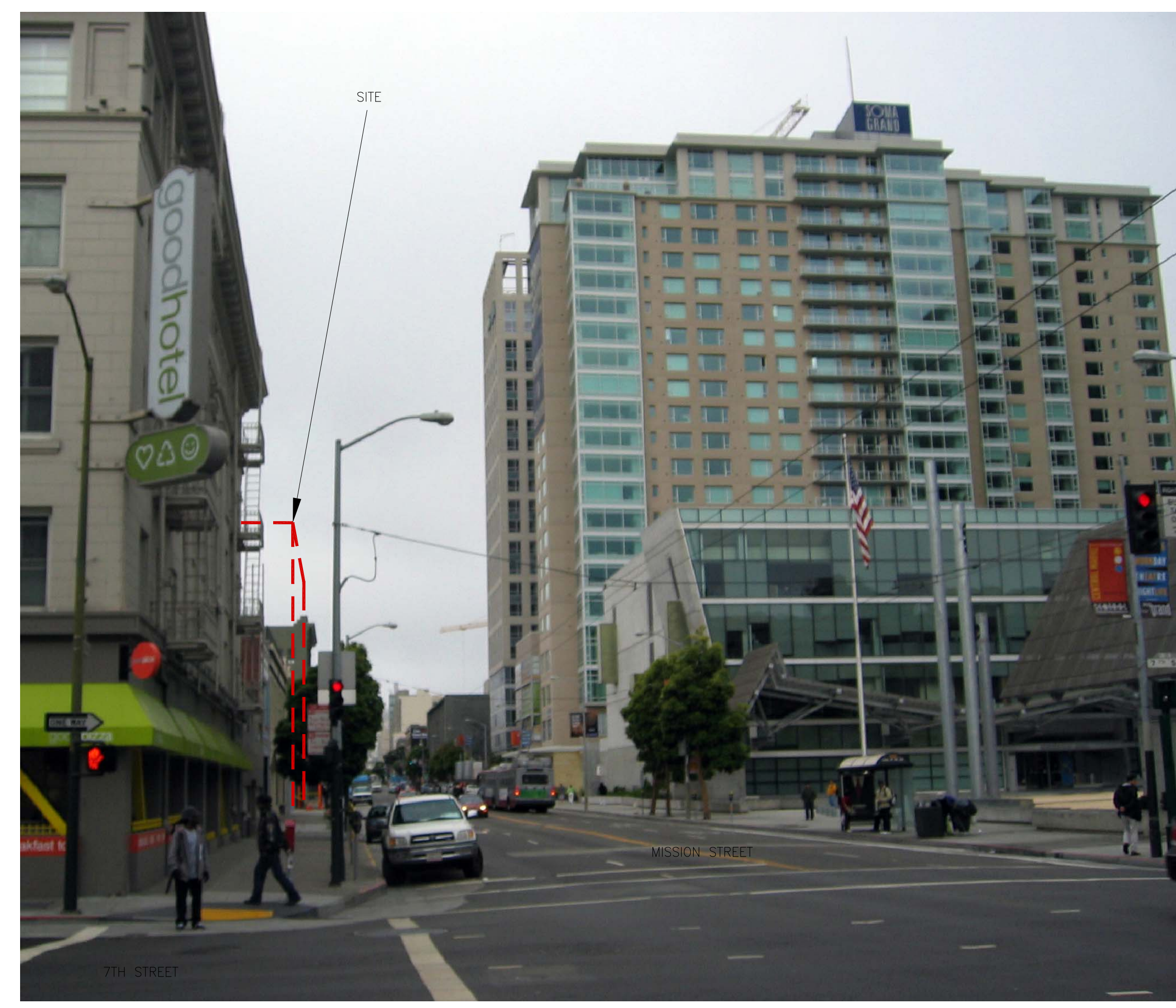
3 BUILDINGS ACROSS THE STREET FROM SITE (PHOTO TAKEN FROM 7TH ST AND MISSION ST) N.T.S.
