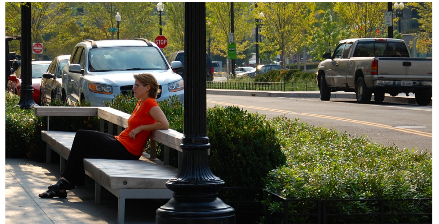
Benches integrated with L.I.D. planters to treat stormwater
