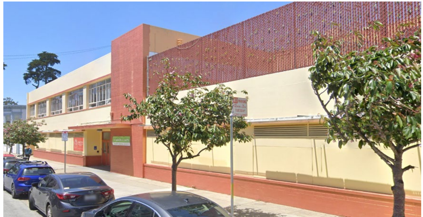
STREET VIEW OF EXISTING SCHOOL STRUCTURE
