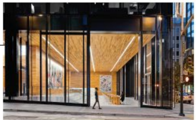
LARGE METAL FRAMED GLASS SLIDING DOORS AT CORNER BUILDING ENTRY
