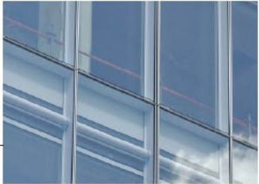
CLEAR GLAZING AT TYPICAL CURTAINWALL AND STOREFRONT
