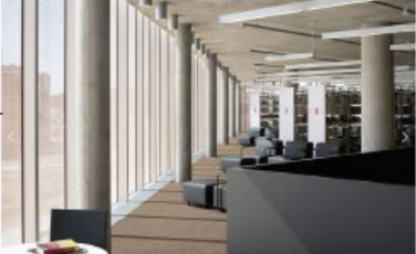
CLEAR GLAZING W/ EXPANDED METAL INTERLAYER PROVIDES SOLAR PROTECTION WHILE ALLOWING VIEWS OUT
