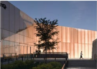
UNITIZED CURTAIN WALL W/ EXPANDED METAL SANDWICHED GLAZING (DARK BRONZE ANODIZED ALUMINUM)
