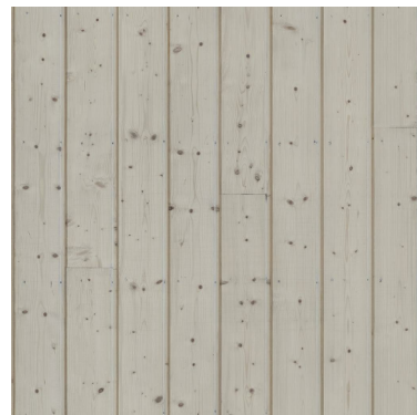
2. VERTICAL WOOD SIDING, STAINED
