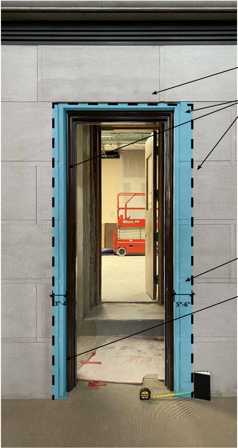
Existing Connection - Area of Demolition
