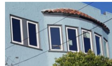
DIVERSE WINDOW TYPES 744 MOULTRIE ST BLDG NORTH
