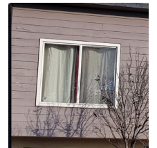
DIVERSE WINDOW TYPES 519 CRESCENT AVE EAST BLDG
