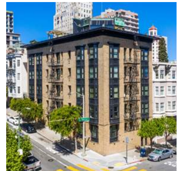
MARK HOPKINS APARTMENTS 1200 SACRAMENTO ST.
