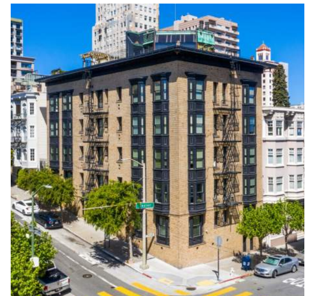
MARK HOPKINS APARTMENTS 1200 SACRAMENTO ST.
