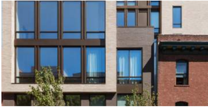
FULL HEIGHT WINDOW IN PROJECTED FRAME
